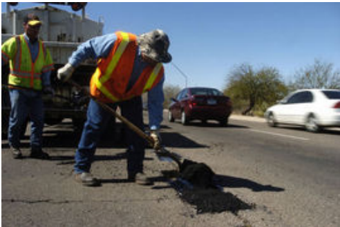
City Streets employees repair potholes on Ward III streets.
