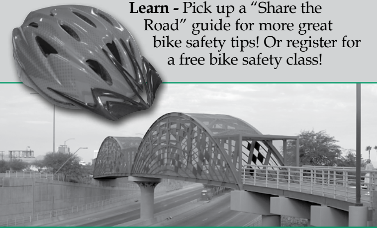
The 'Basket Bridge' over Euclid Avenue near Park Avenue offers pedestrians and cyclists a continuous nine-mile path from downtown Tucson to Escalante Road and Kolb Road.
