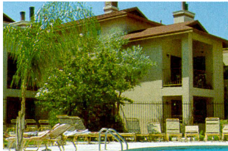
Apartments are convenient to employment centers, shopping, and recreation.
