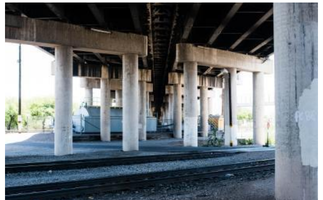
Existing 22nd Street Bridge, view of railroad tracks under bridge
