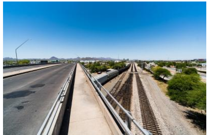
Existing 22nd Street Bridge, view over railroad tracks
