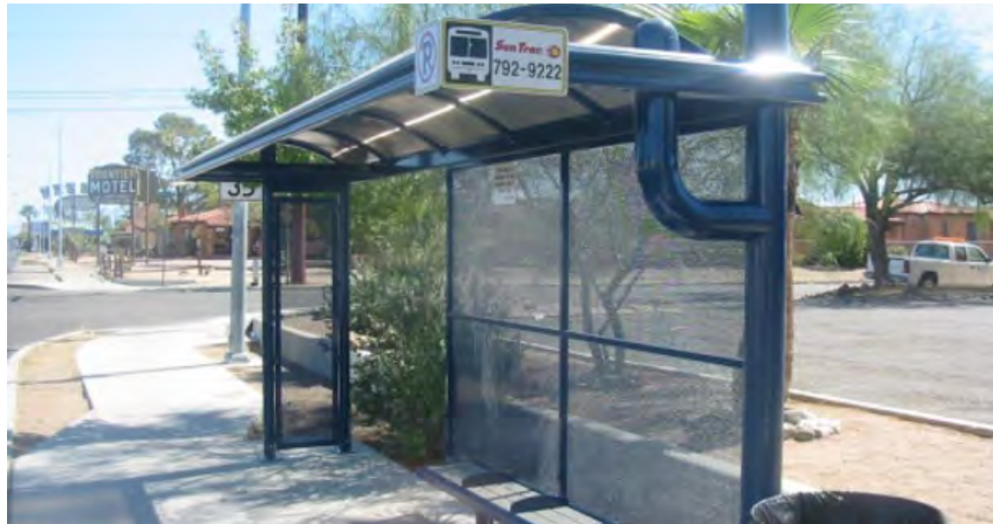
▲ Recycled, customized bus shelters with seating and solar lighting installed on east and west sides of Oracle Road.
