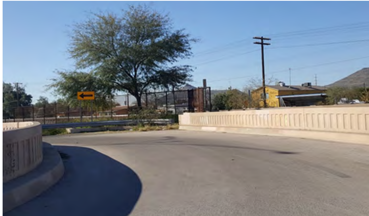
▲ Concept 1: Underutilized Vehicular Overpass on Speedway (Current Condition)
