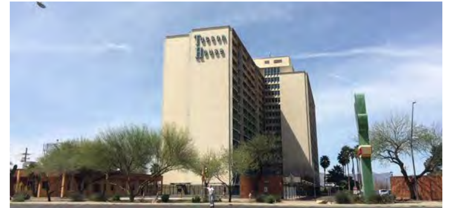
▲ Tucson House stands alone as the only high-rise housing in the area.
