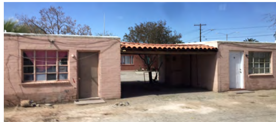
▲ Some motor courts and casita villages suffer from disinvestment and neglect.
