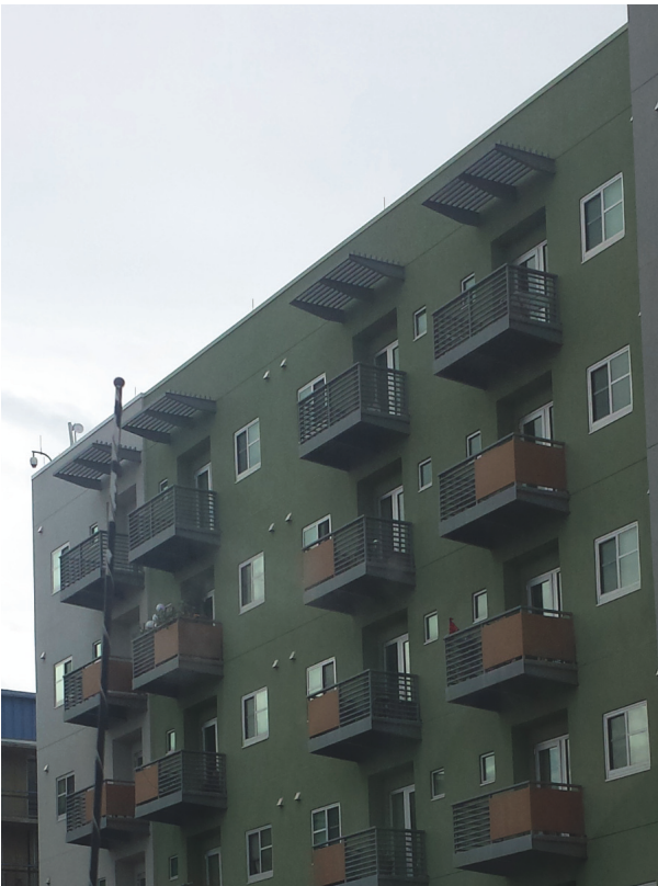
MLK Apartments 55 North 5th Avenue, Tucson, AZ 85701
