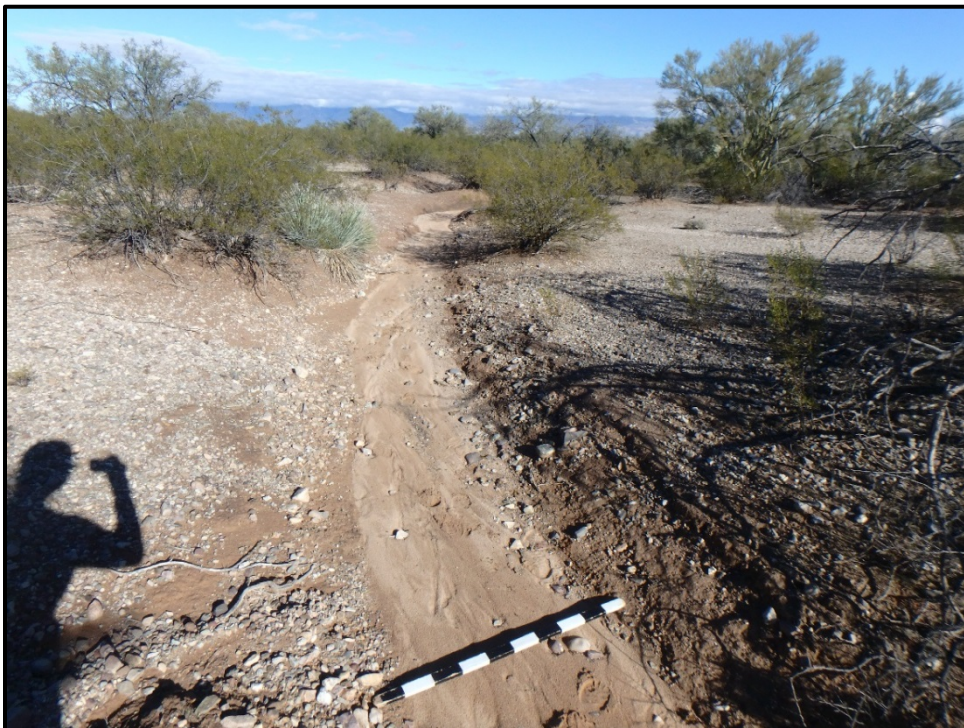
Photo 10. An overview of PP-5, a swale in the project area.
