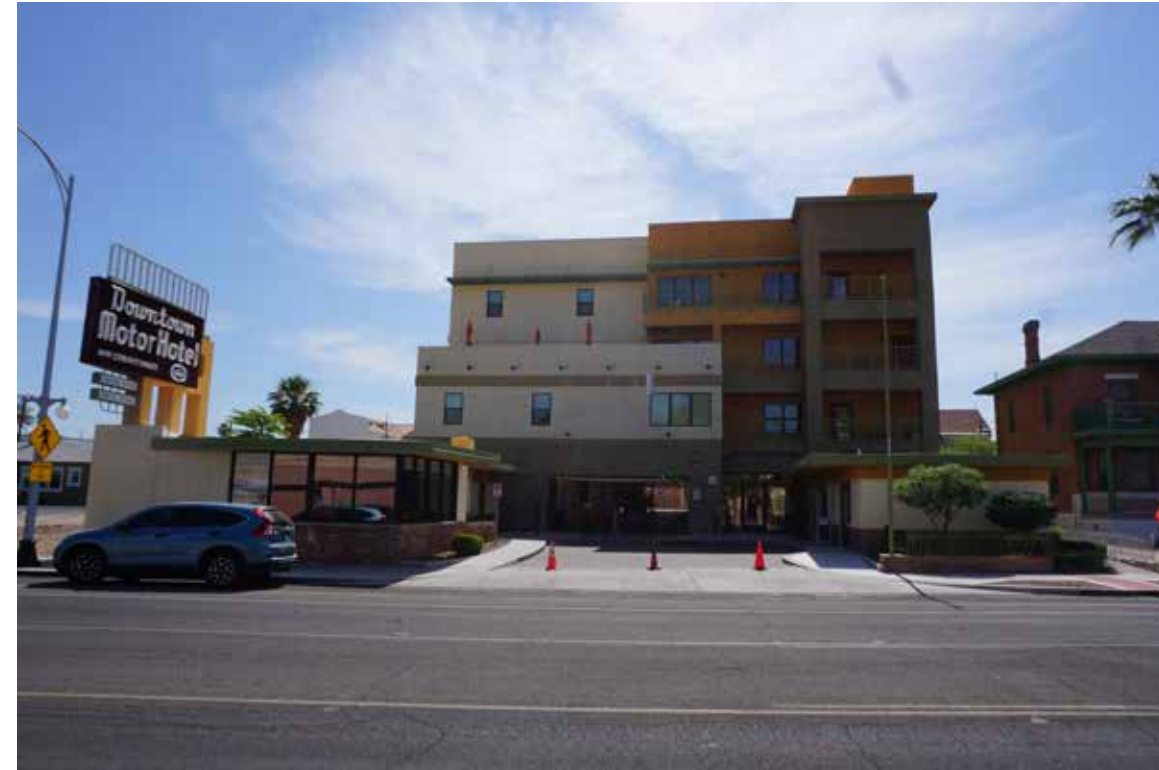
383 SOUTH STONE AVENUE CONTIBUTING - NATIONAL DISTRICT ONLY
