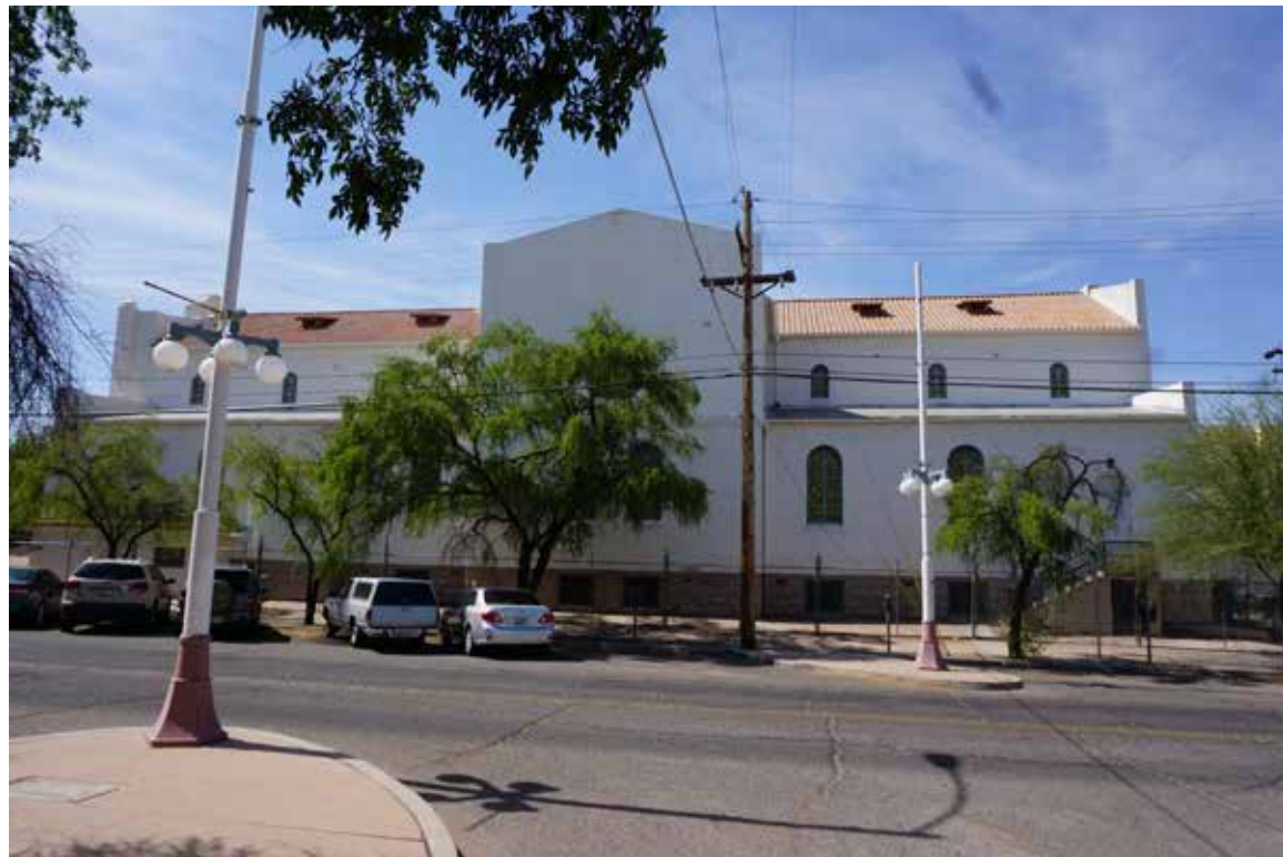
408 SOUTH 6TH AVENUE CONTIBUTING - LOCAL AND NATIONAL DISTRICT
