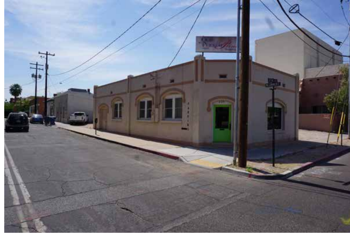
255 SOUTH STONE AVENUE CONTIBUTING - NATIONAL DISTRICT ONLY
