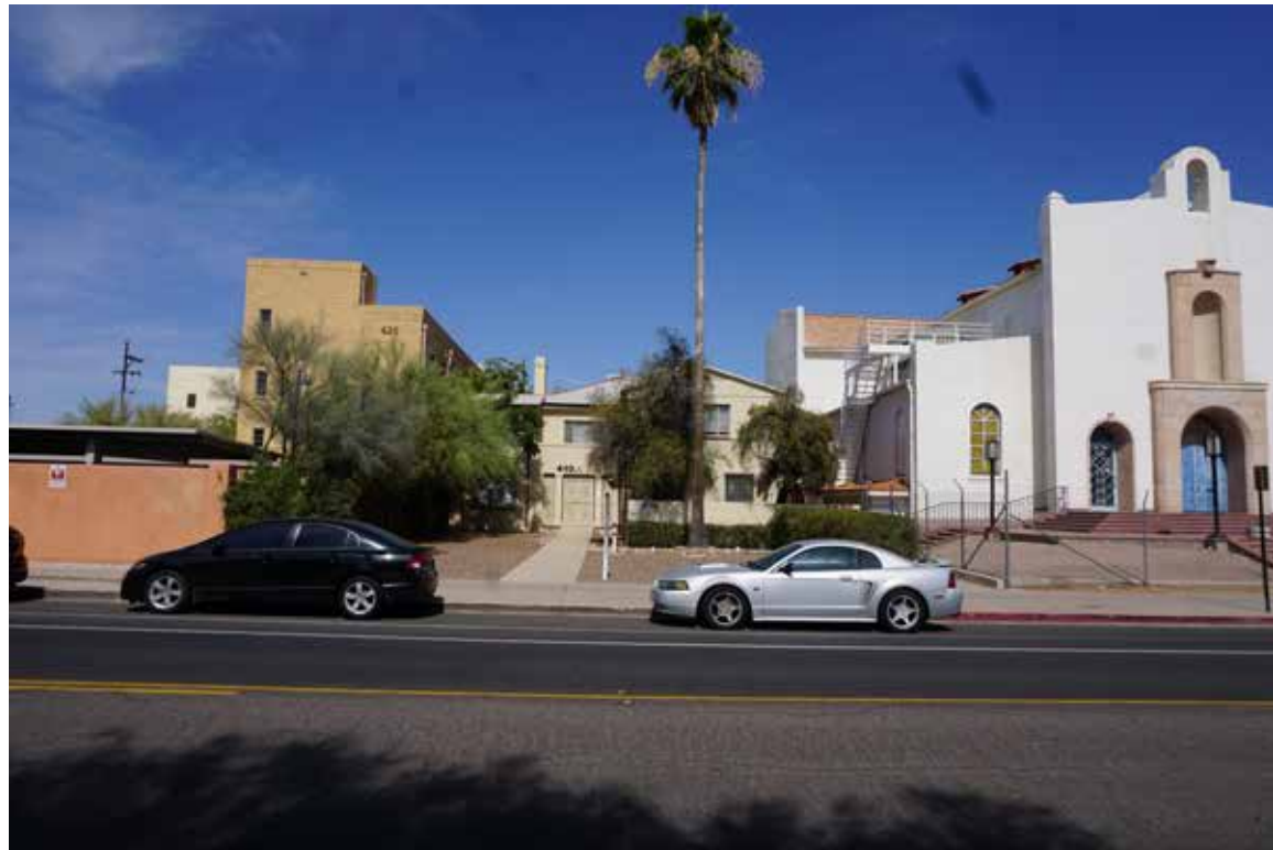
410 SOUTH 6TH AVENUE CONTIBUTING - LOCAL AND NATIONAL DISTRICT
