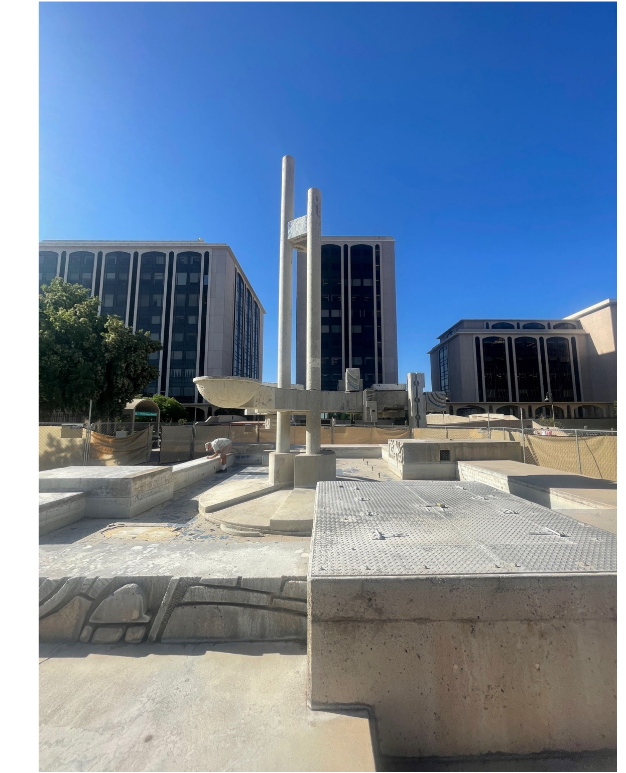
OVERALL FOUNTAIN - VIEW FROM NORTH
