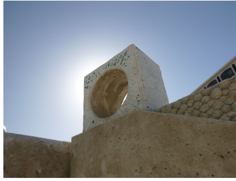
DECORATIVE BLOCK 7 NORTH-WEST
