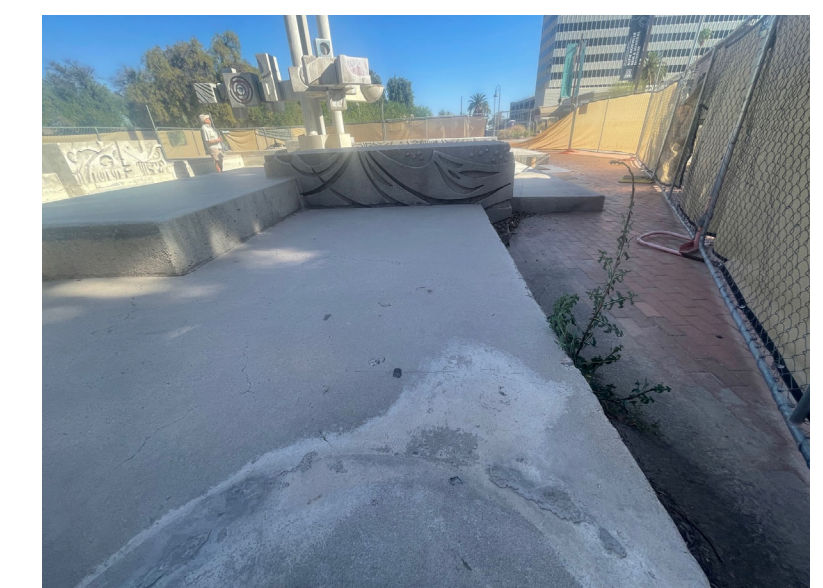
SOUTH-WEST CORNER CONDITION
