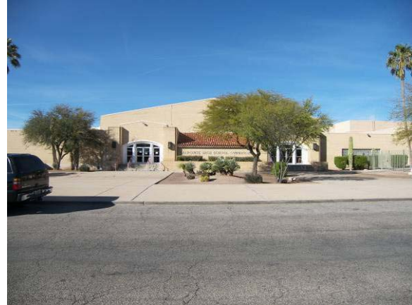
Photo 2: Looking north across Copper at the gymnasium.
