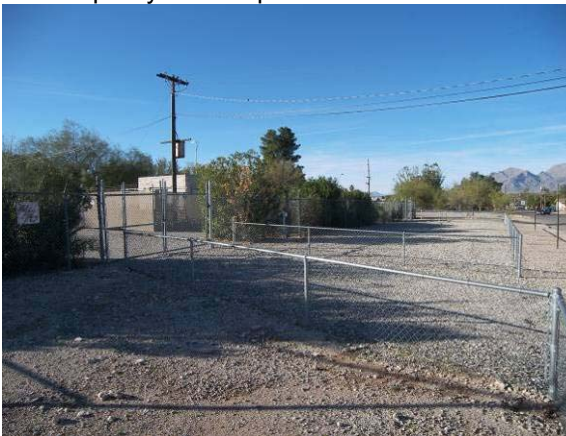
Photo 17: Looking north at the Tucson Water Facility located along Copper.
