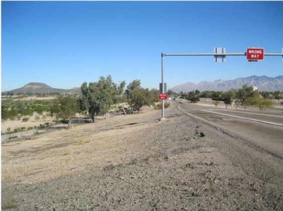
PHOTO 6: NORTH ON I-19
