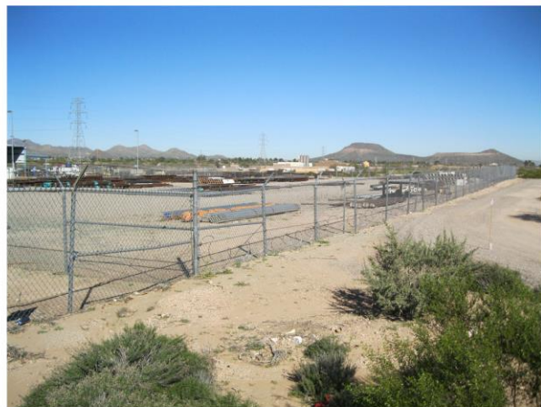
PHOTO 11: VIEW TO NORTHWEST FROM IRVINGTON
