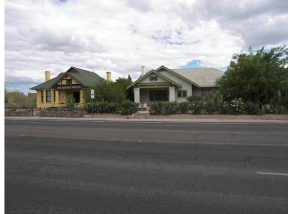
Photo 2: Single-family bungalows along Speedway typical of the areas architecture.
