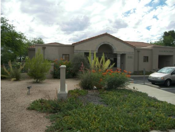
Photo 1: Looking at the front entrance of Kelsch from 4th Avenue.
