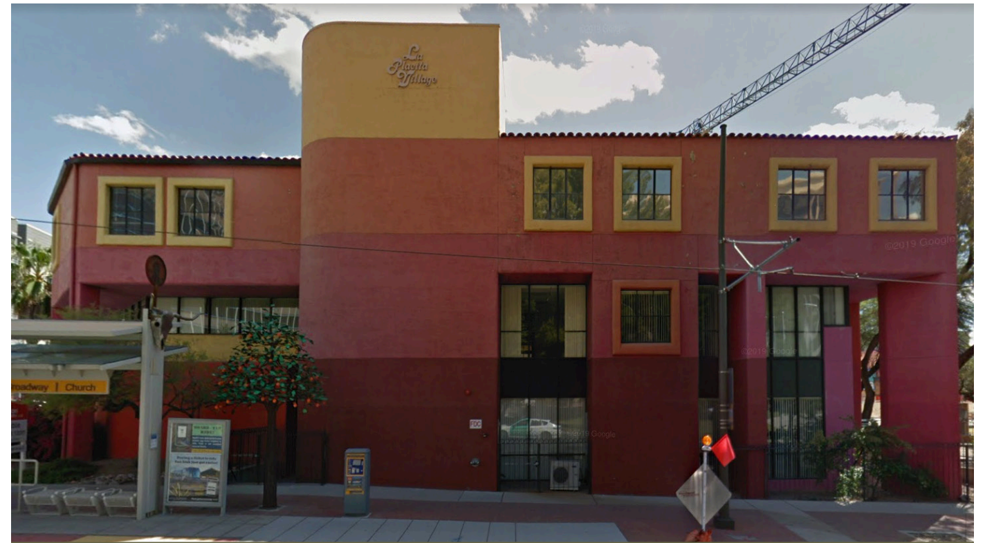
A | PHOTOGRAPH : EXISTING VIEW FROM BROADWAY
