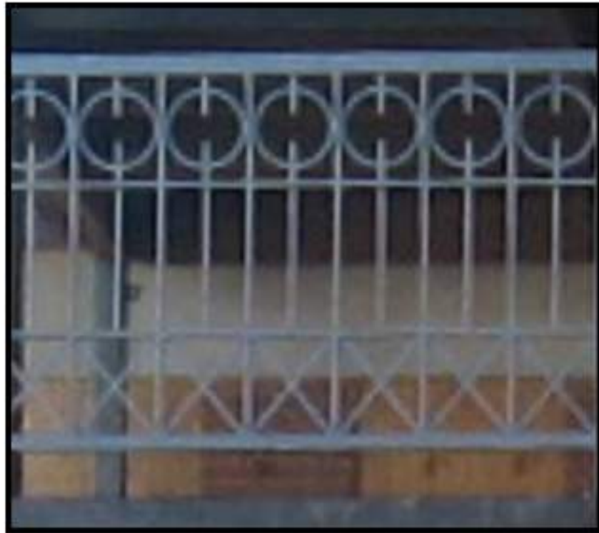
NEW GAURD RAIL PAINTED PER OWNER COLOR BY DUNN EDWARDS Formal Gray DE6382 RL#594
