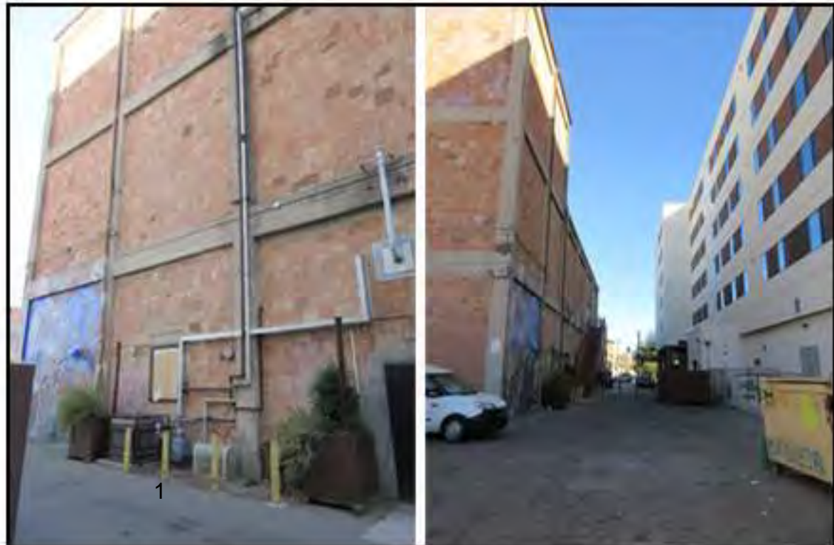
SOUTHEAST CORNER AND ALLEY LOOKING NORTH
