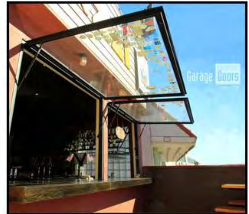
OPERABLE AWNING WINDOWS OPERATIONAL SAMPLE
