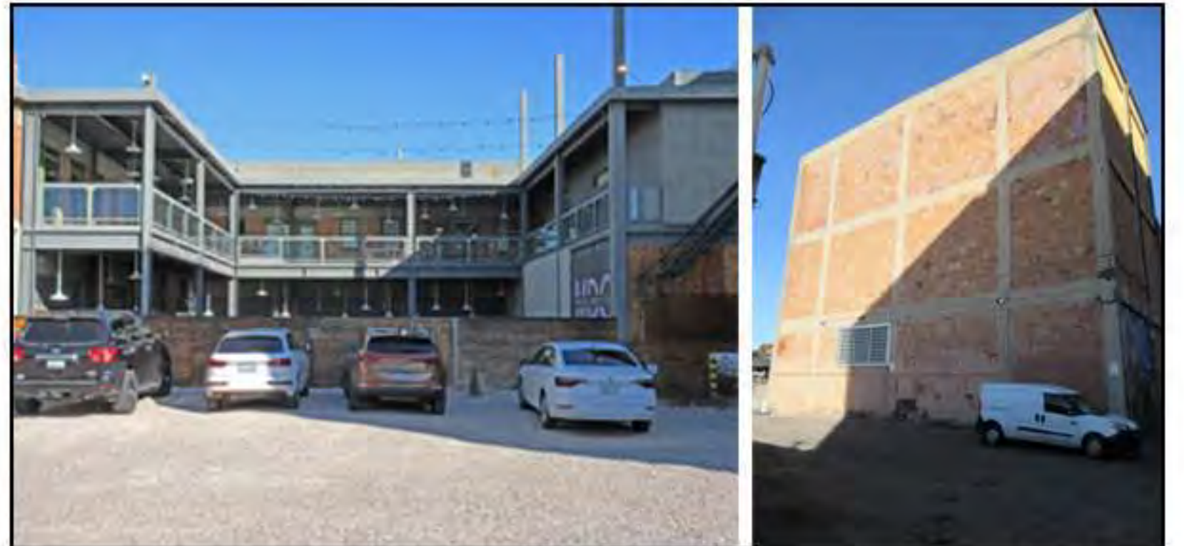
ELEVATION LOOKING NORTH AND SOUTHEAST CORNER
