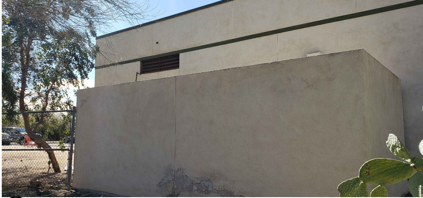
EAST ELEVATION PHOTO SCALE: NTS
