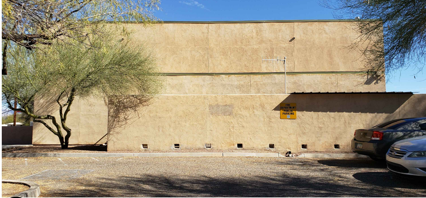
WEST ELEVATION PHOTO SCALE: NTS
