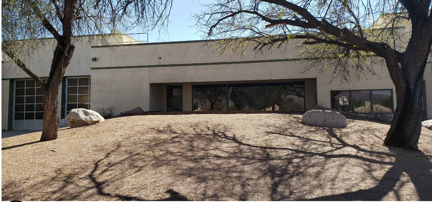
NORTH ELEVATION PHOTO SCALE: NTS
