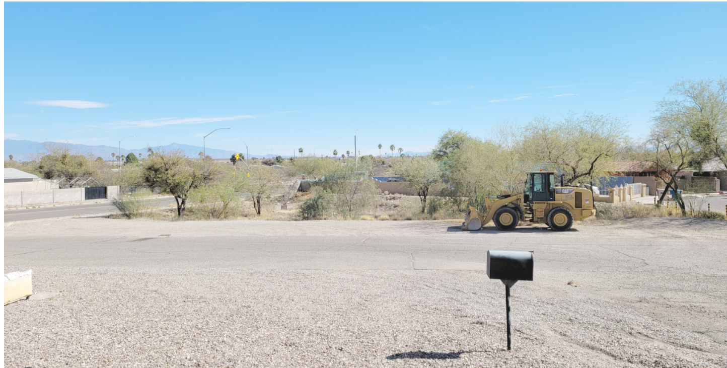
VIEW LOOKING SOUTH/SOUTHEAST SCALE: NTS
