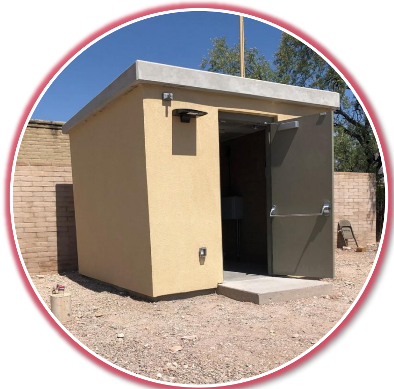
CONTROL BUILDING (100 SF)
