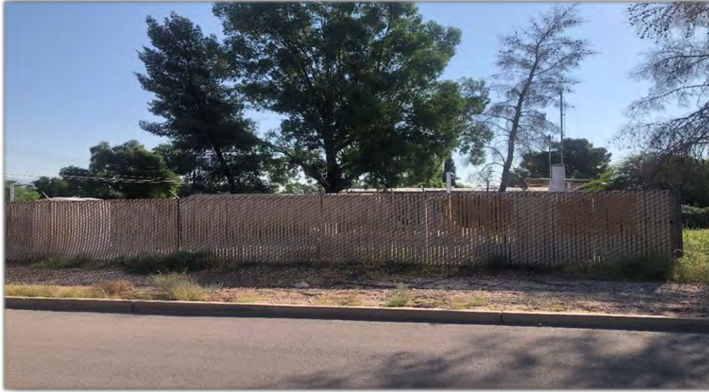
Existing screening around the entire perimeter of the well yard.
