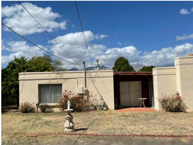
EXHIBIT #19 (Adjacent property to the North)
