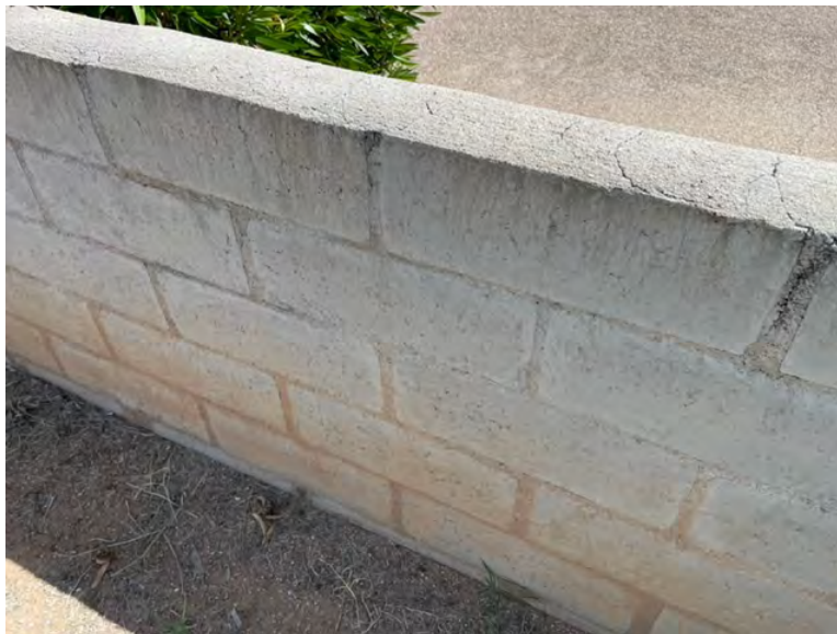
EXHIBIT #7 (Close up- Southern Site Property Wall-West Section)
