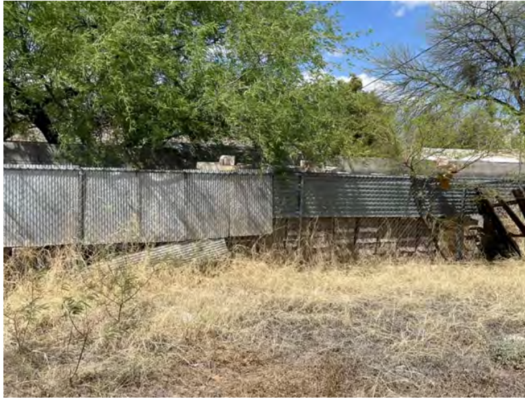
EXHIBIT #14 (Existing North-West Corner of the property with corrugated metal fence to be replace by block wall)
