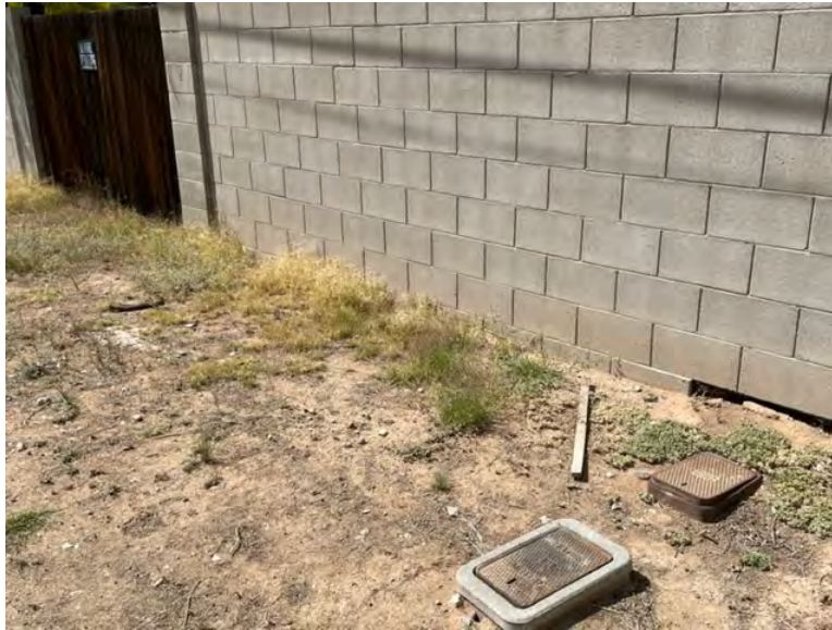
EXHIBIT #20 (Existing Water Meter adjacent to North Site Wall with in the Easement)
