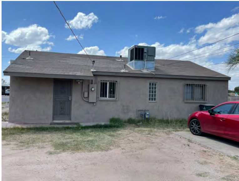
EXHIBIT #4 (Rear-West Elevation of Existing Building)
