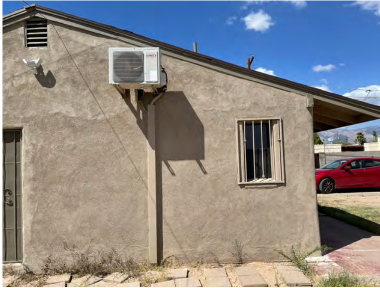
EXHIBIT #3 (Side-South Elevation of Existing Building-East Section)
