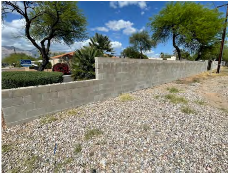
EXHIBIT #29 (Northern Property Wall- West Section)
