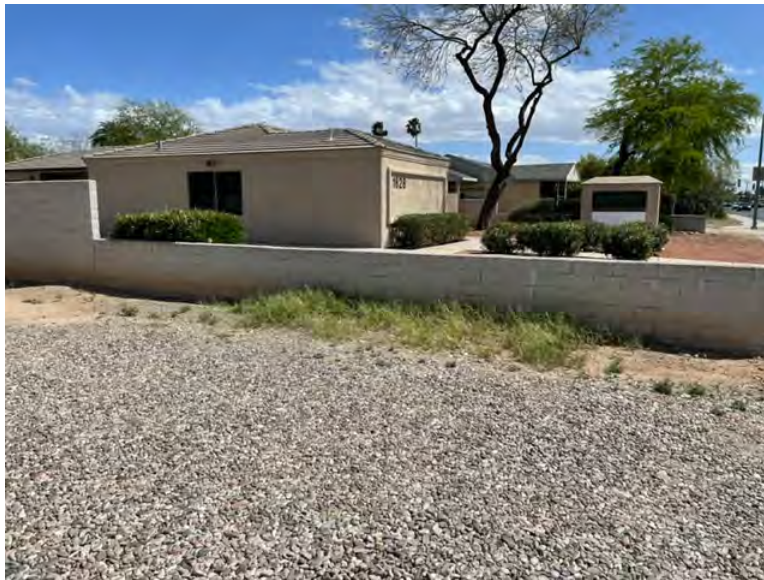
EXHIBIT #5 (Southern Site Property Wall-West Section)
