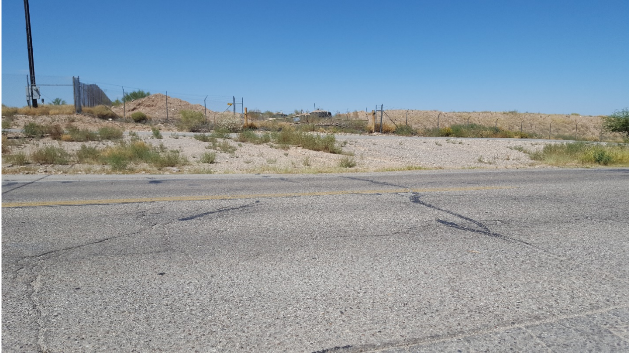
Photo 2: Existing entrance at southeast corner of property. Not viable for public entry.
