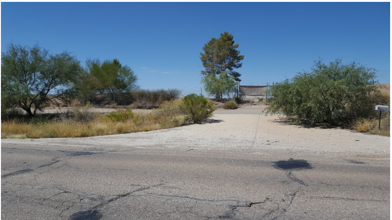
Photo 5: Existing Harrison Rd entrance to be improved and used by the public.
