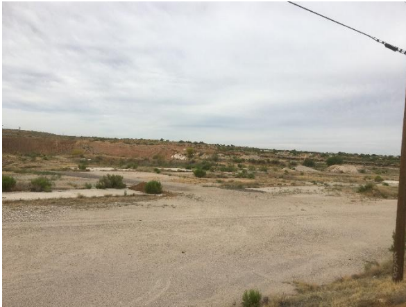
Photo #1 View of concrete slabs remaining from mine operations in Area A.
