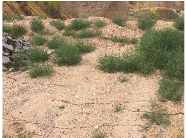
Photo #4 Stress Cracks along fill edge in Area B.
