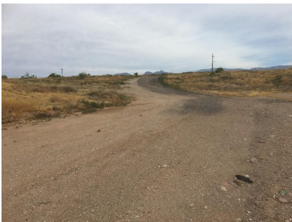
Photo #5 View of existing road within Area A2.
