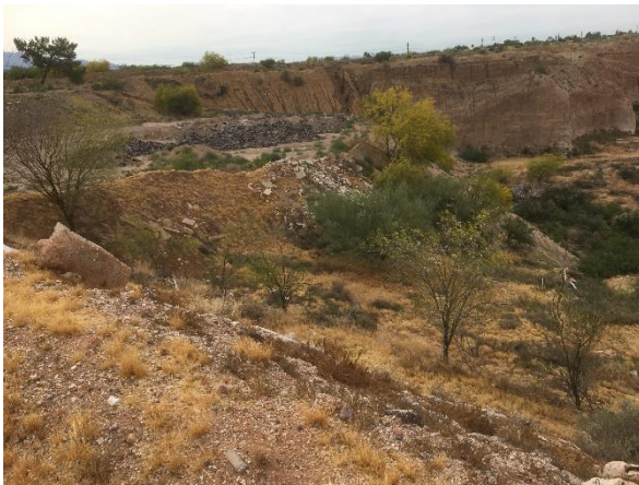
Photo #3 Side view of fill area and debris within Area B.
