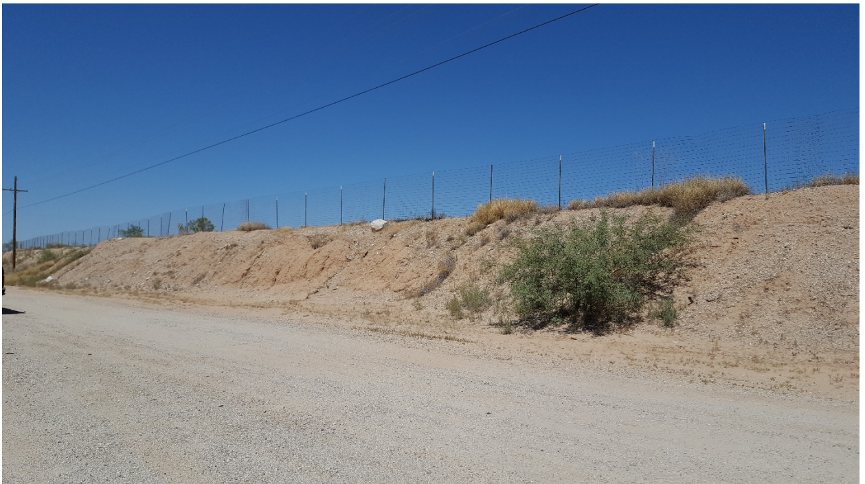
Photo 9: View from within the property (north part). Looking northwest. Pantano Wash on opposite side of berm.
