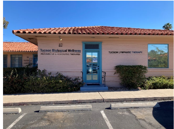
Photo 15: Looking east at building near southeast corner of Property.
