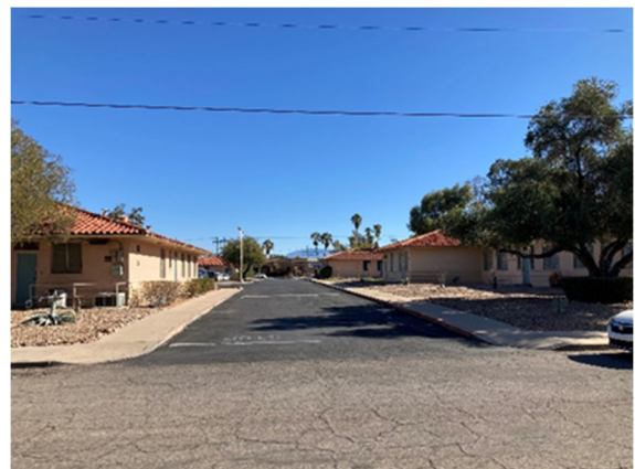
Photo 4: Looking east at central access drive through Property from its intersection on Norton Ave.
