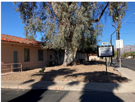
Photo 9: Looking north along Tucson Blvd. from Property's southernmost access drive.
