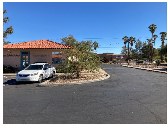
Photo 17: Looking east toward Tucson Blvd. at southern access from parking lot.
