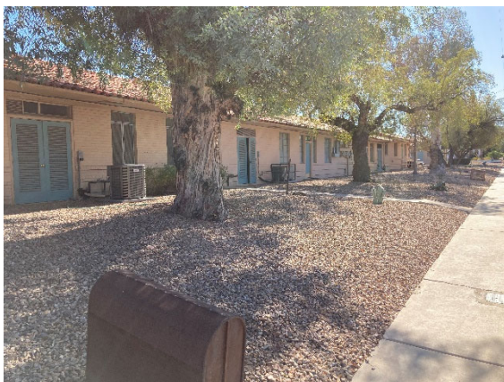
Photo 3: Looking southeast at Property from sidewalk along Norton Ave.
