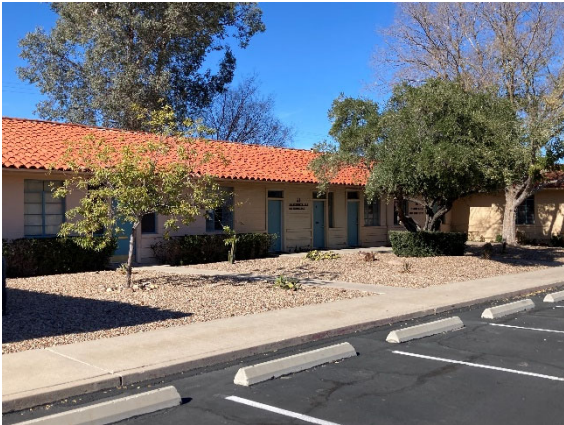
Photo 22: Looking northwest at building in southwest corner of Property.
