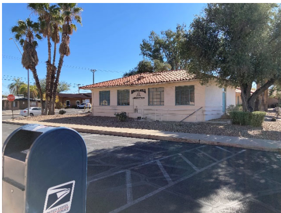
Photo 16: Looking southeast at building near central access at Tucson Blvd. from parking lot.
