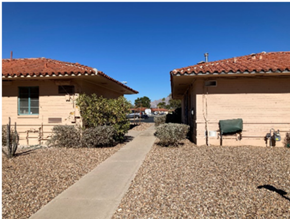
Photo 7: Looking south at pedestrian access into Property from Adams St.
