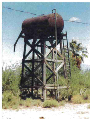
Water tank at Esmond Station
