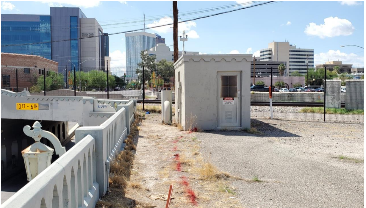
Figure 25. North elevation of pump house, Parcel Number 117-05-068F
