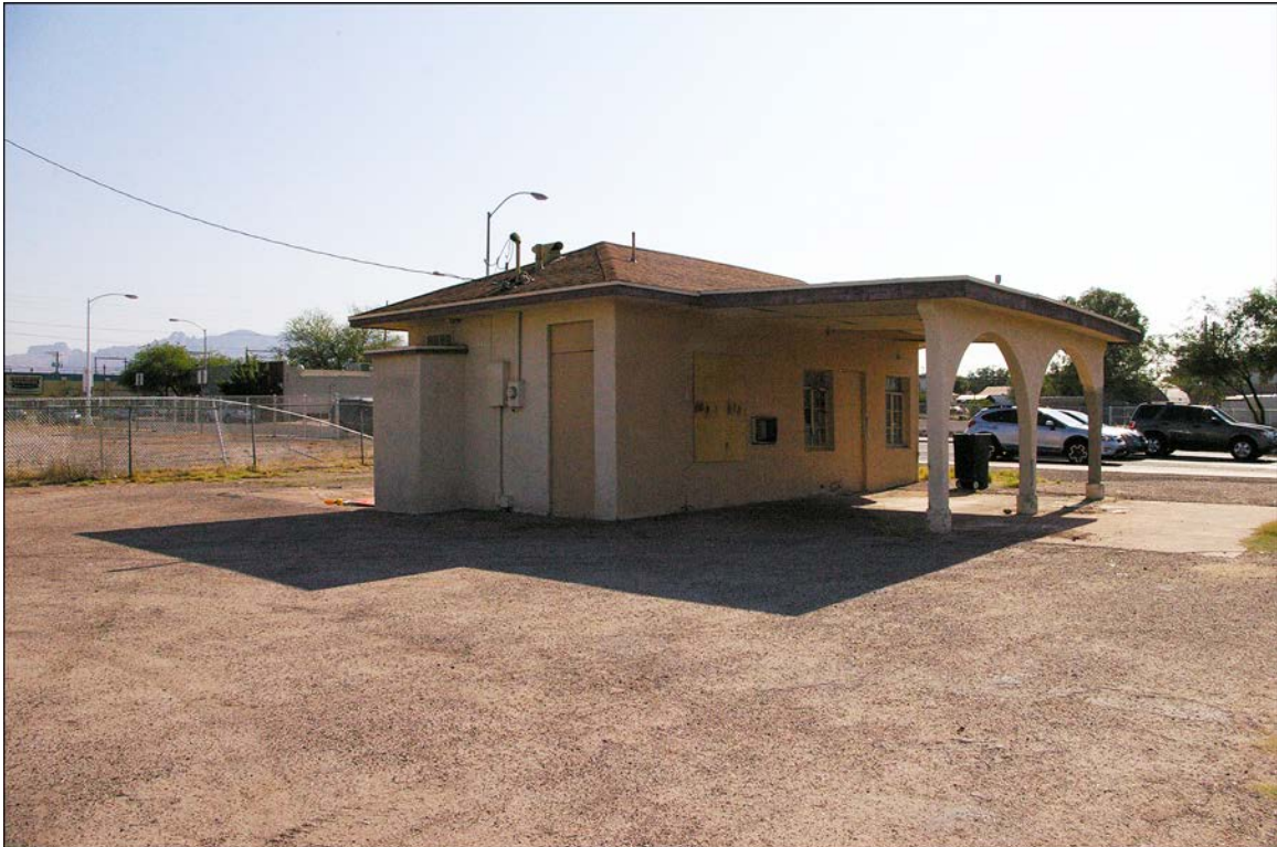
Figure 7. South and west elevations of main building, 503 North Stone Avenue.
