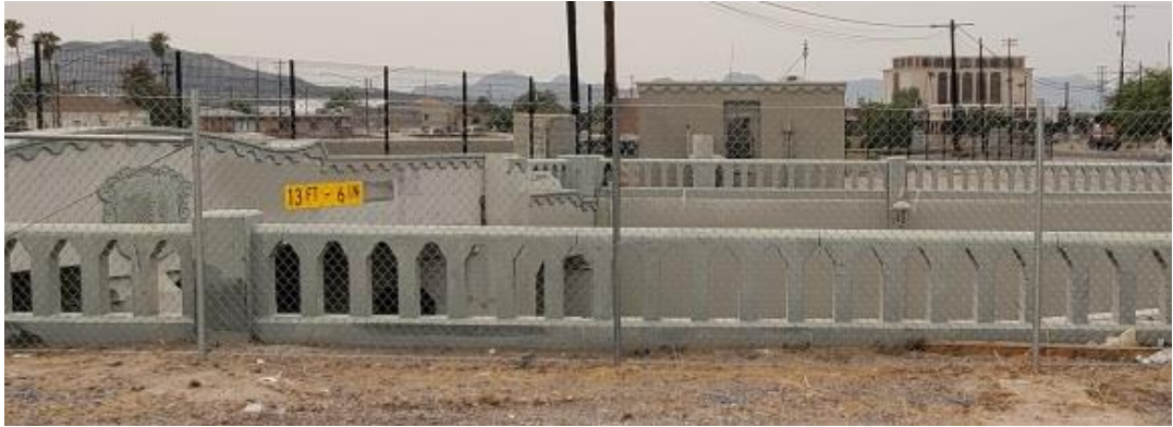
Figure 29. East elevation of pump house, Parcel Number 117-05-068F
