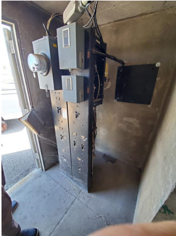
Figure 30. Interior, south west elevation of pump house, Parcel Number 117-05-068F
