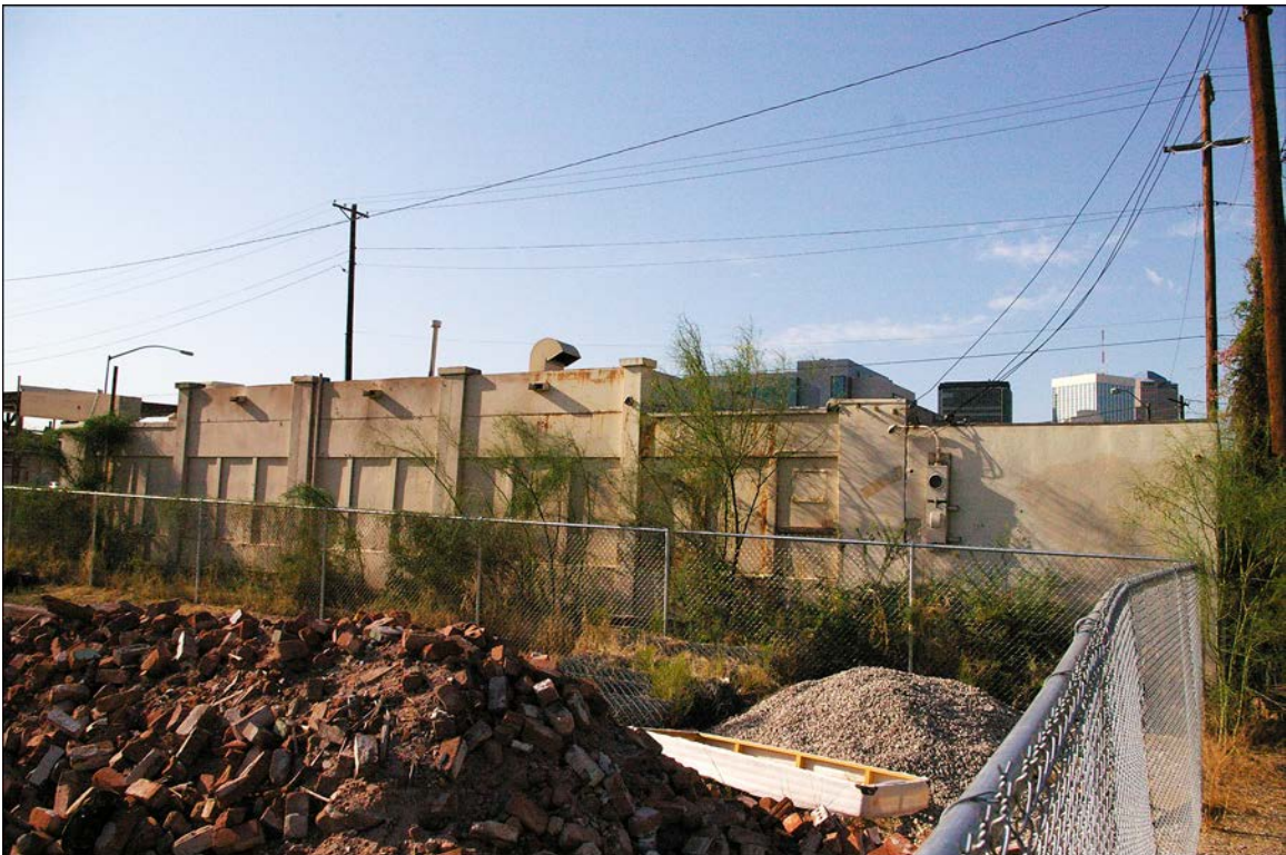
Figure 13. North elevation of service building, 503 North Stone Avenue.
