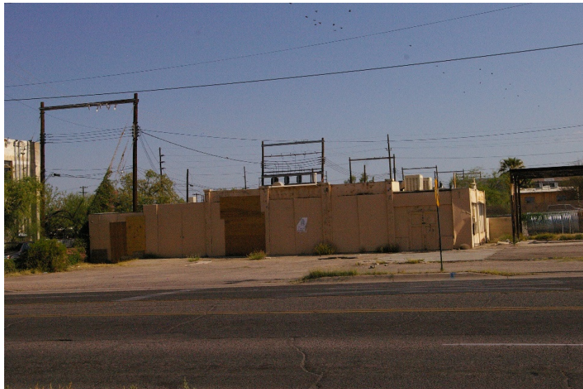
South elevation of service building, 503 North Stone Avenue.
