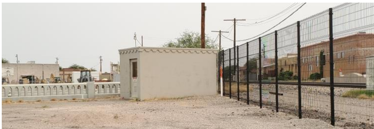
Figure 26. West elevation of pump house, Parcel Number 117-05-068F
