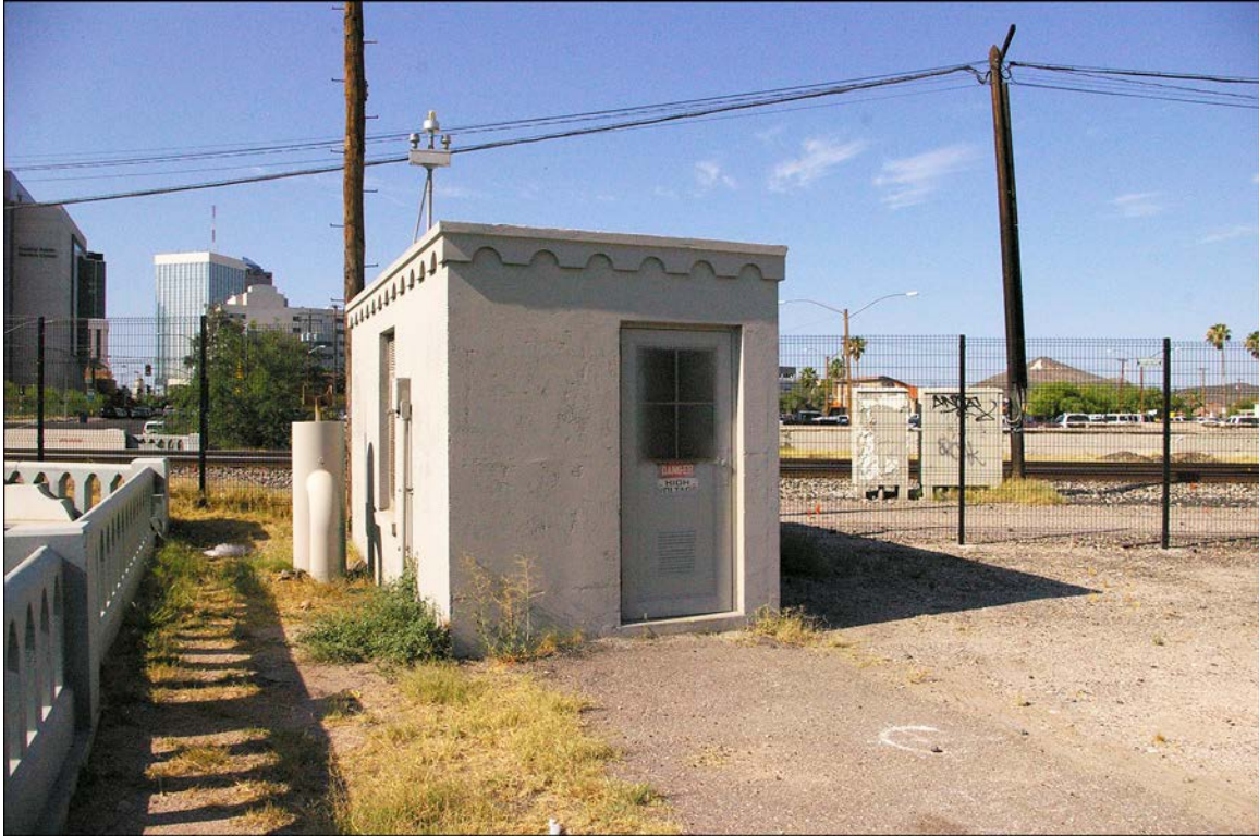
Figure 20. East and north elevations of pump house, Parcel Number 117-05-068F.
