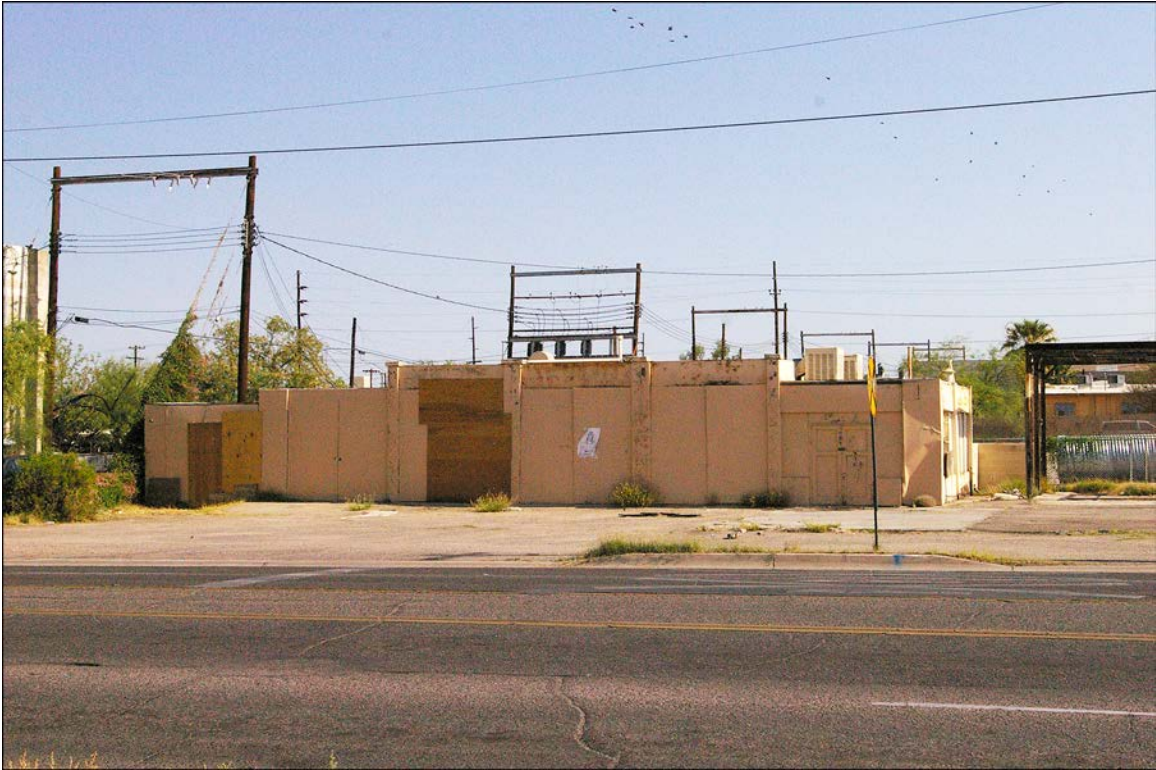
Figure 12. South elevation of service building, 503 North Stone Avenue.
