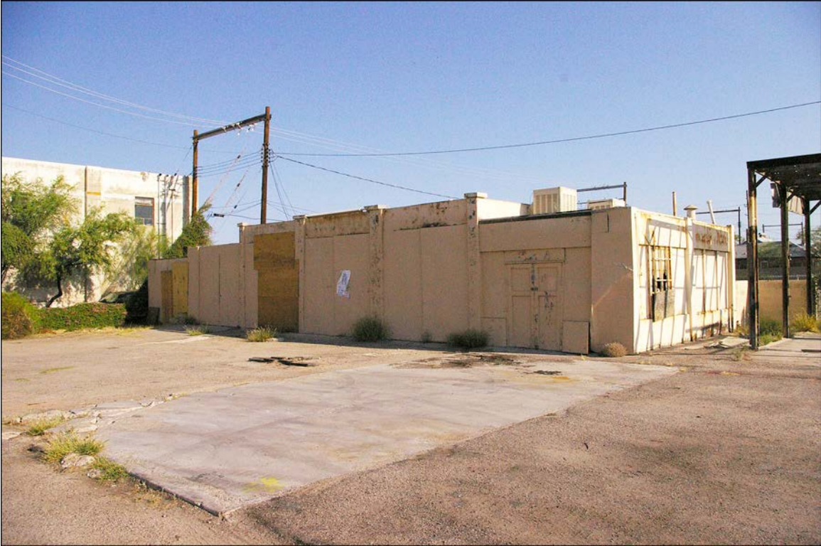
Figure 14. South and east elevations of service building, 503 North Stone Avenue.
