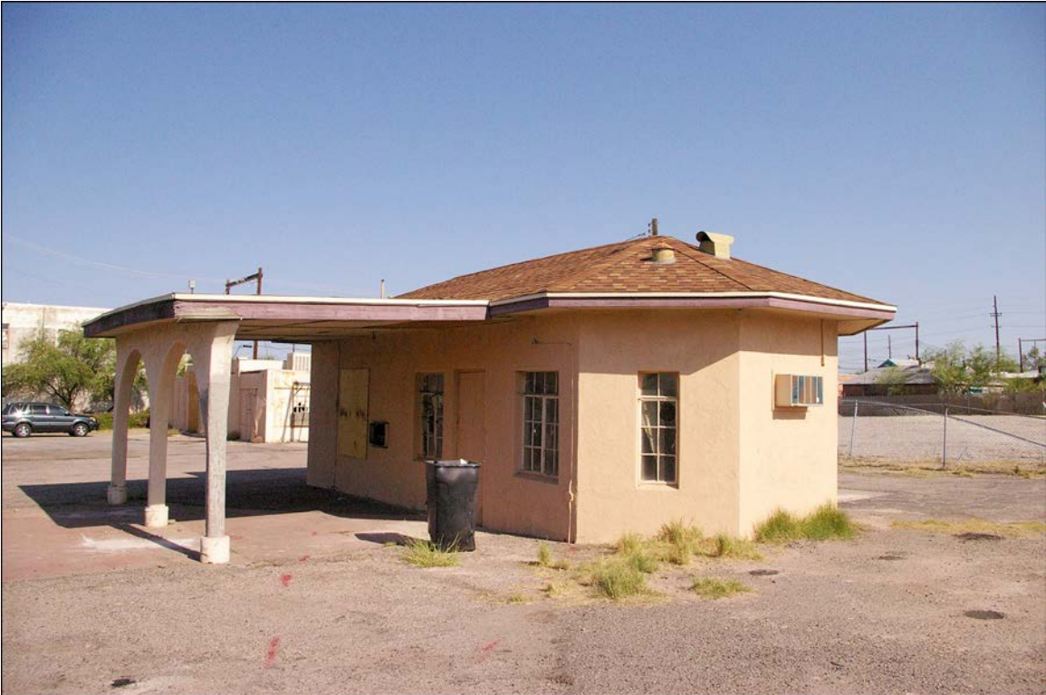
Figure 5. South and east elevations of main building, 503 North Stone Avenue.
