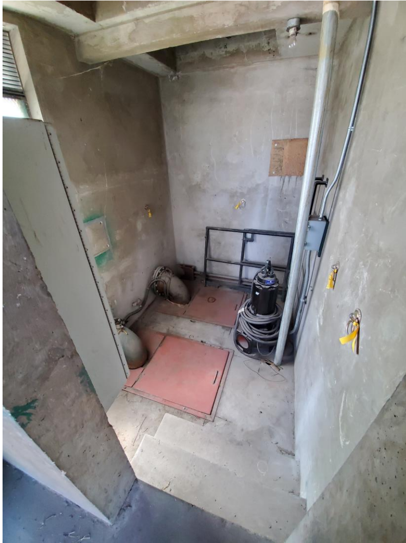
Figure 32. Interior, north west elevation of pump house, Parcel Number 117-05-068F
