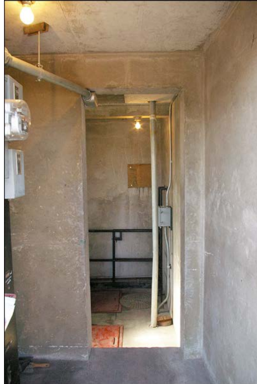
Figure 23. Interior of pump house, Parcel Number 117-05-068F; view to the south.
