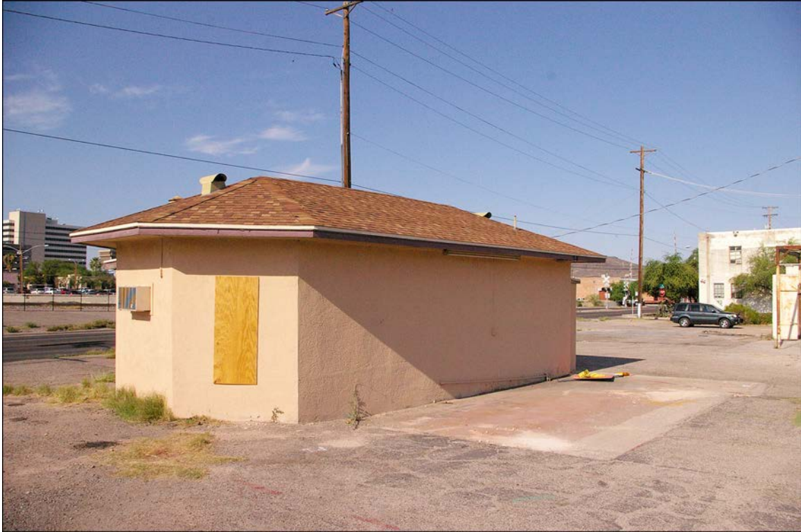
Figure 6. East and north elevations of main building, 503 North Stone Avenue.
