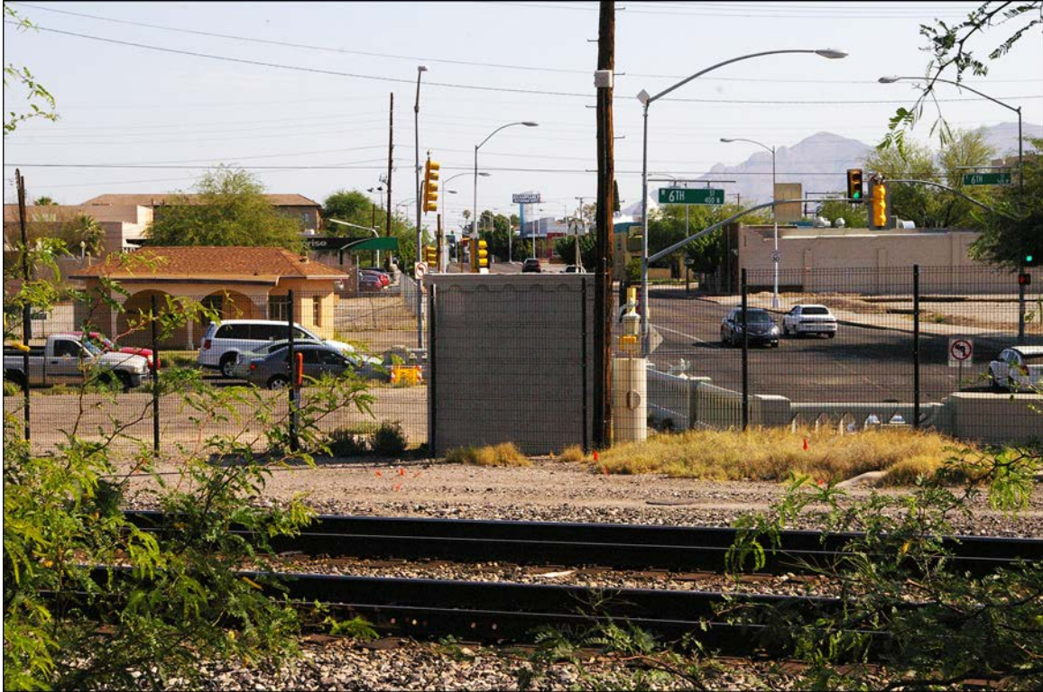
Figure 22. South elevation of pump house, Parcel Number 117-05-068F.
