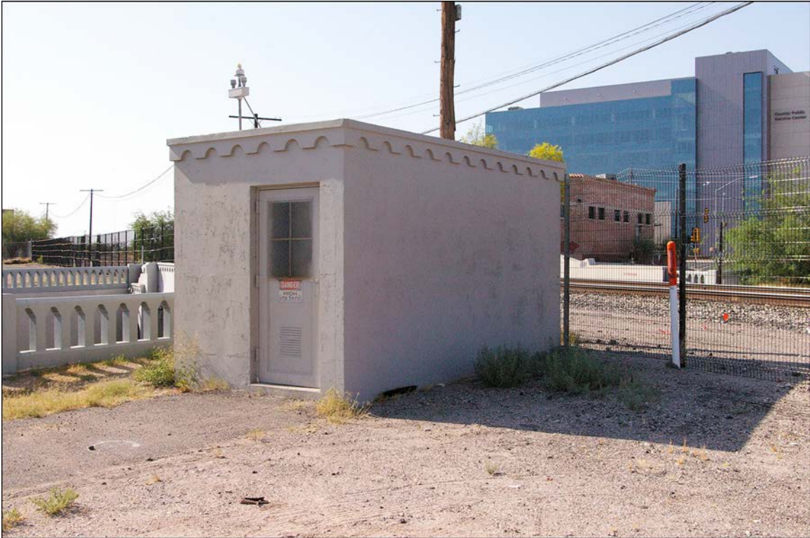
Figure 21. North and west elevations of pump house, Parcel Number 117-05-068F.
