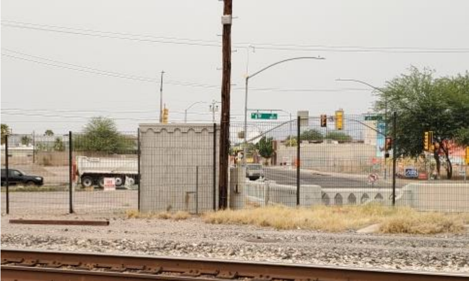
Figure 27. South elevation of pump house, Parcel Number 117-05-068F
