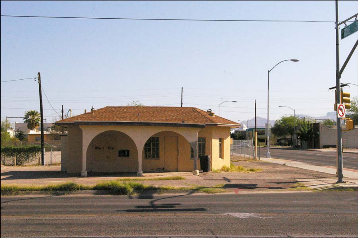
Figure 4. South elevation of main building, 503 North Stone Avenue.
