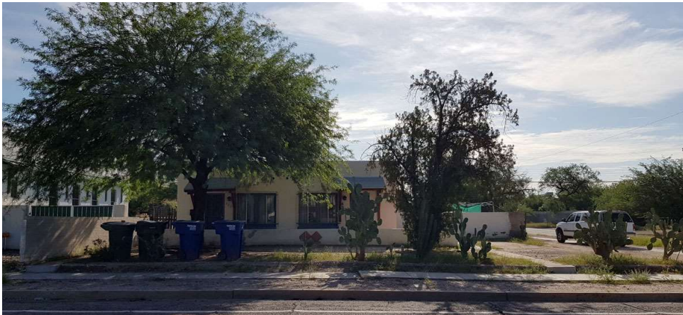
West – front facing 4 th Avenue
