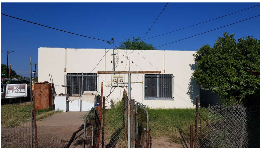
East – rear facing Railroad Avenue
