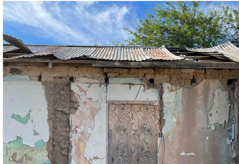
CORRUGATED GALVANIZED METAL ROOF
