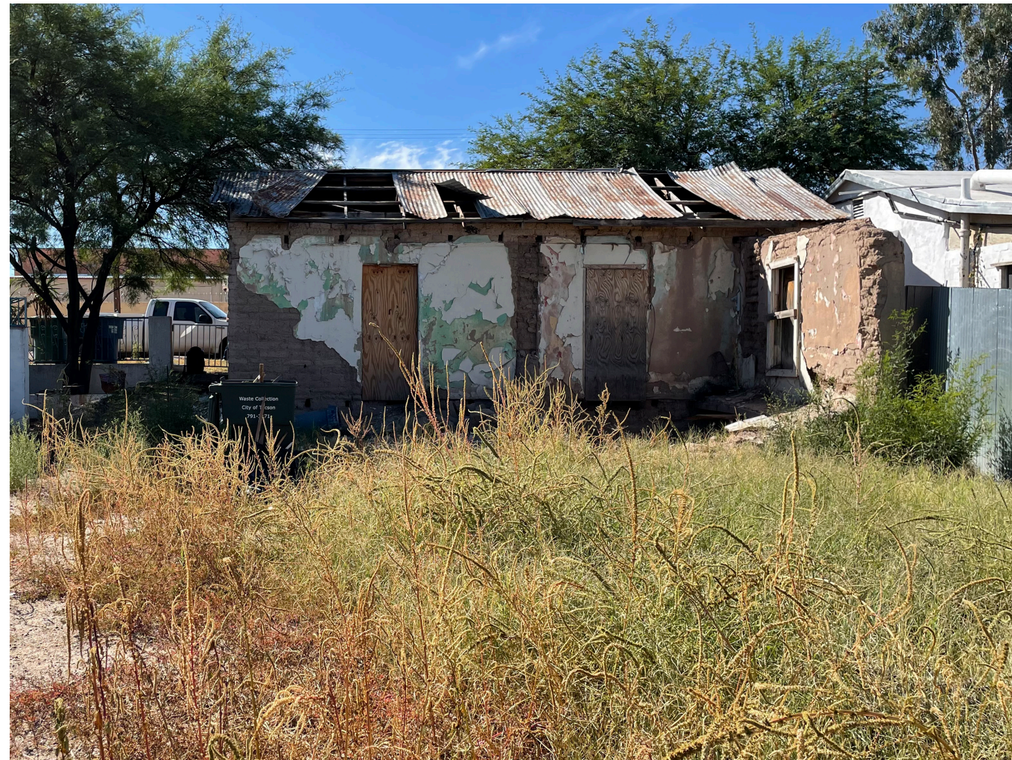
NORTH ELEVATION (ALLEY)
