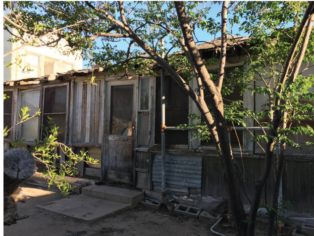
NORTH VIEW OF EXISTING PORCH TO BE REMOVED
