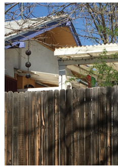
13 Example of wood and polycarbonate shed porch addition
