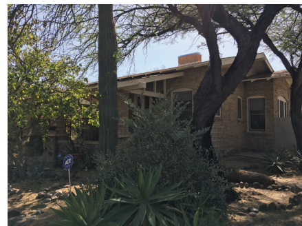
8 Example of shed form porch below eave of main house
