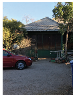
10 9 Example of material change between porch and main house and openings with vertical proportions
