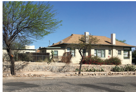
7 Example of shed porch below eave
