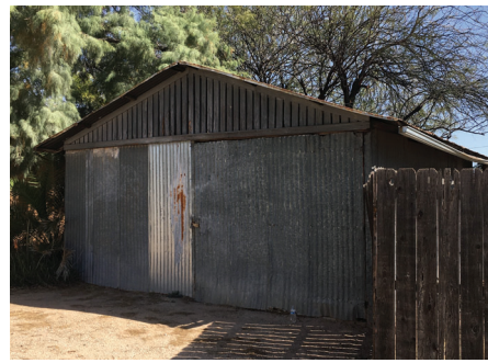
12 11 Examples of vertical slatted wood over corrugated siding
