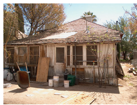
View of rear porch to be removed
