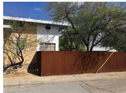
4 Example of material change at porch addition and weathering steel
