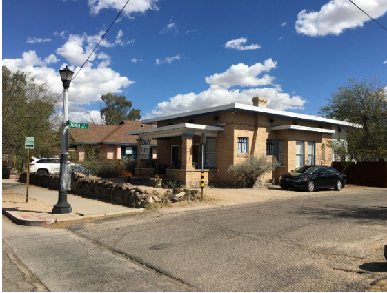
628 E. 5 th St. example of additive porch form
