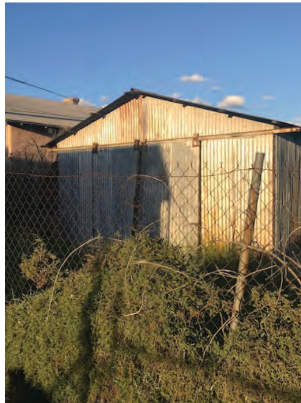
827 S HERBERT - CONTRIBUTING GALVANIZED CORRUGATED METAL SIDING
