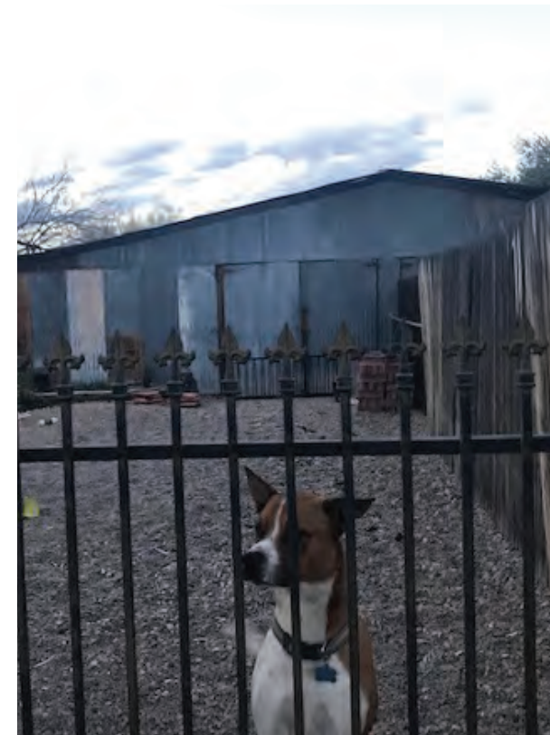
847 S 5TH AVE- CONTRIBUTING GALVANIZED CORRUGATED METAL SIDING
