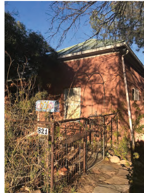
821 S 5TH AVE - CONTRIBUTING STANDING SEAM ROOF
