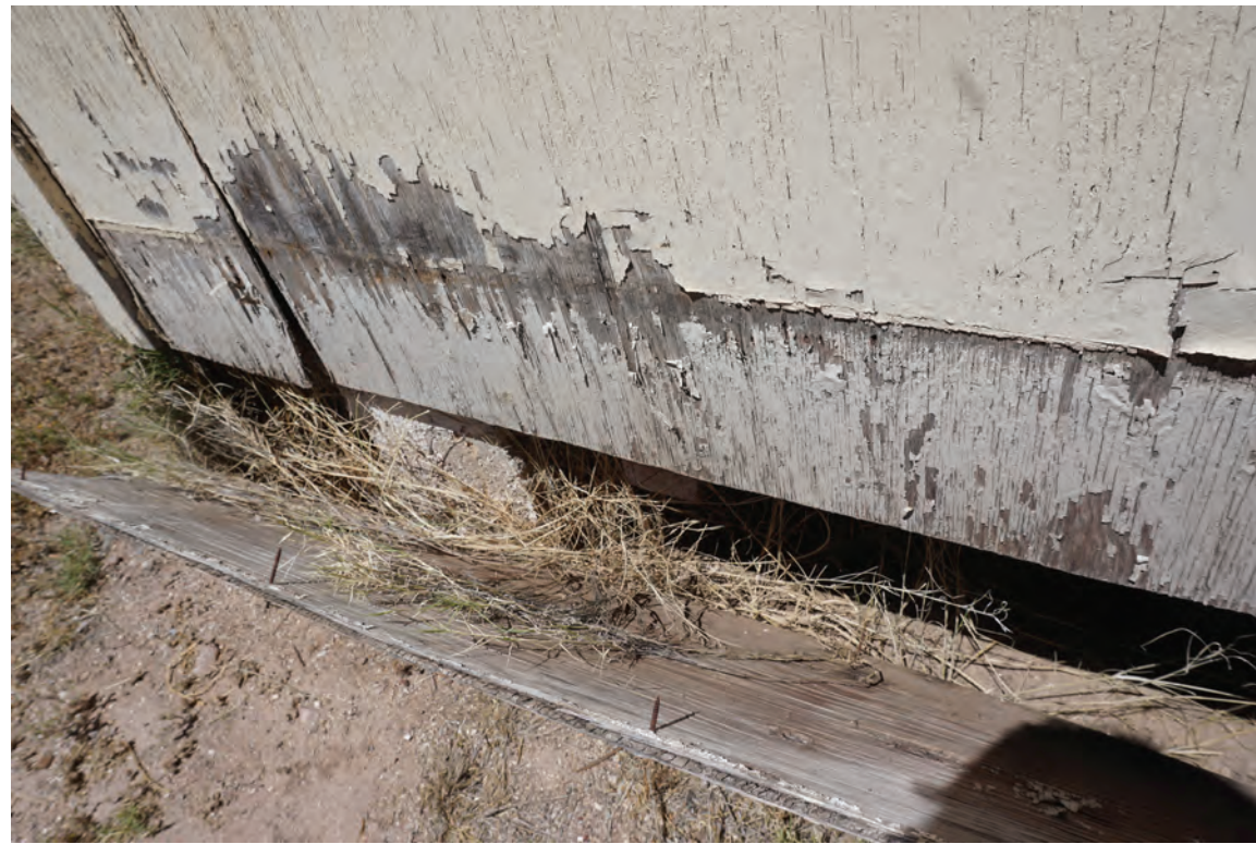
PORCH SUPPORT, SOUTHWEST CORNER
