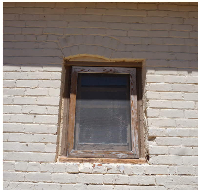
SOUTH ELEVATION, MIDDLE WINDOW
