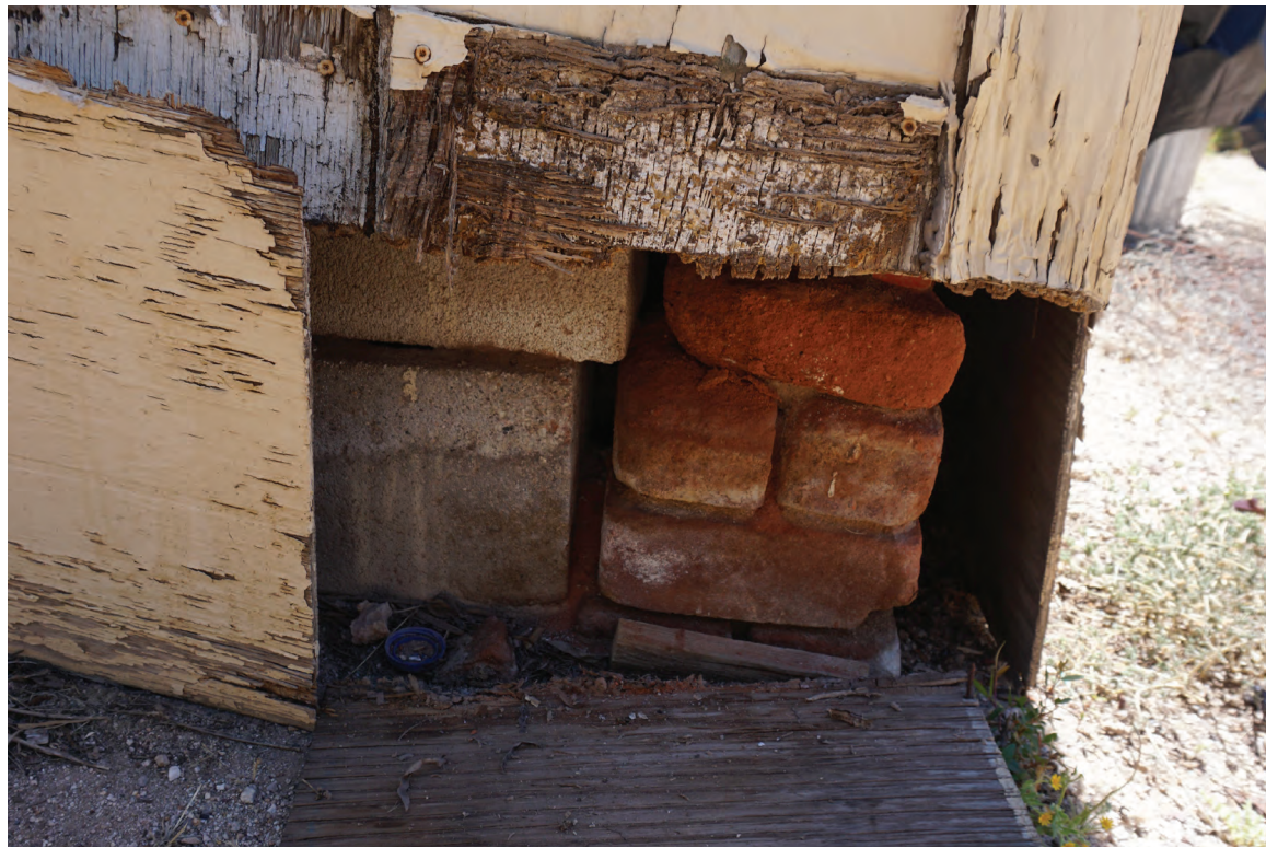
PORCH SUPPORT, NORTHWEST SUPPORT
