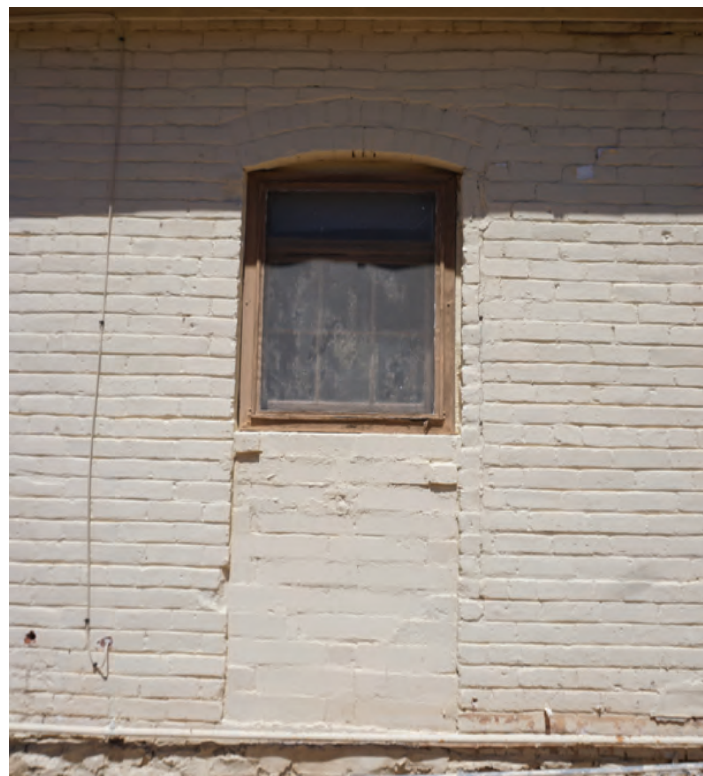
SOUTH ELEVATION, WEST WINDOW
