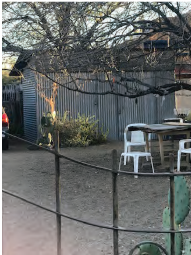
803 S 5TH AVE - CONTRIBUTING GALVANIZED CORRUGATED METAL SIDING
