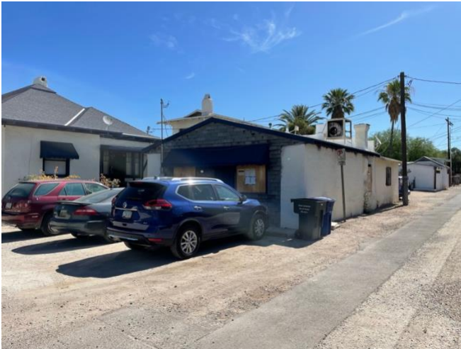
502 E. University building at back of property
