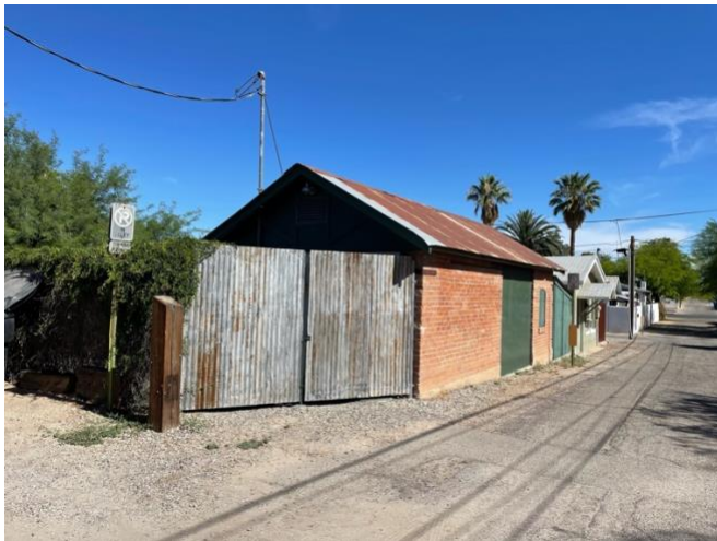
722 N 3 rd building at back of property
