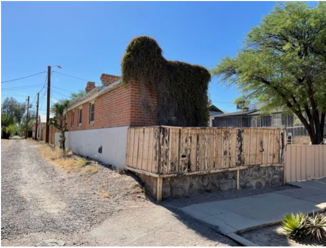
501 E 4 th Ave building at back of property
