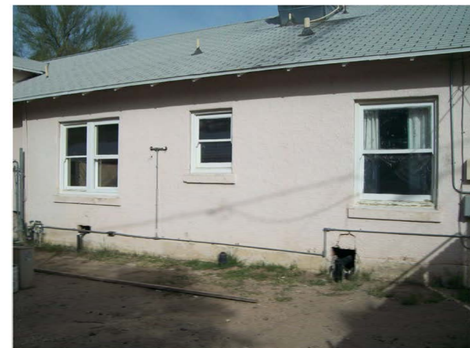
#2 east end of South Wall
