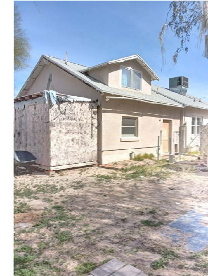
#8 SW corner (Note Unattached plywood shed to be demolished)
