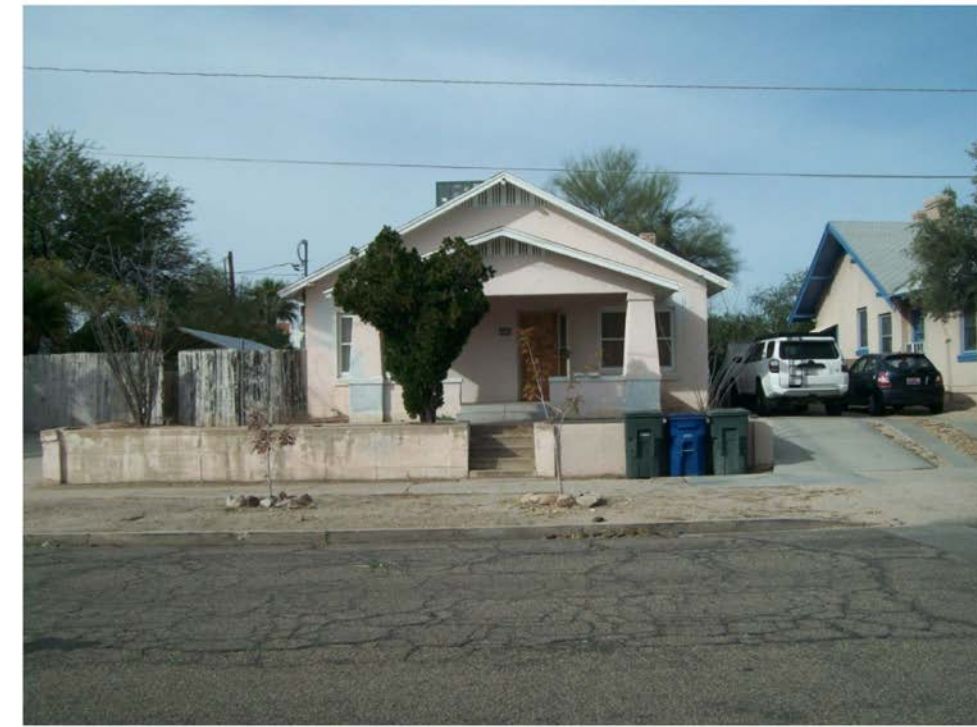
#1 825 N 3 rd Ave East
