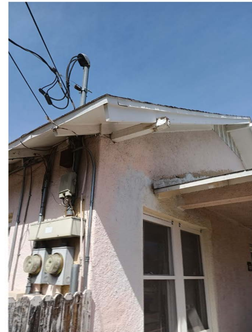
#1 Repair sagging brace
