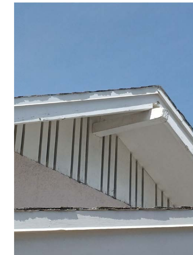
#2 Repair sagging brace
