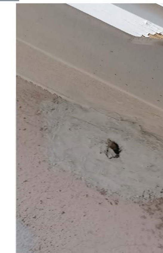
#3 Replace missing brace
