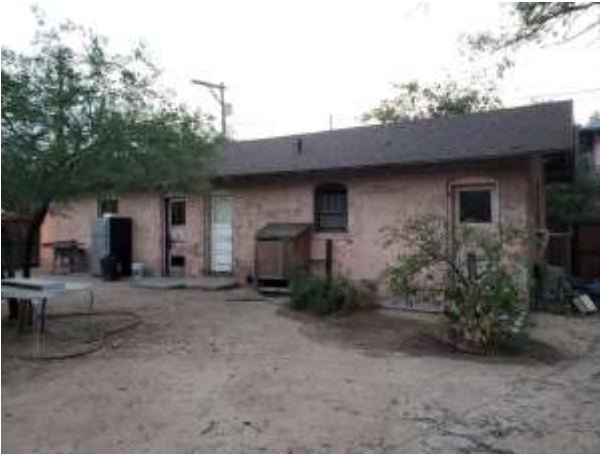
East face north end of guest house
