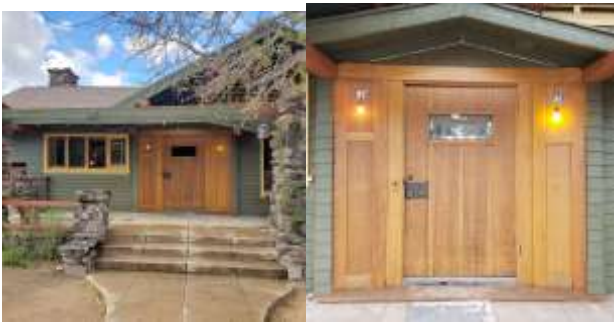
Front entry door after picture: clear polyurethane finish by Behr
