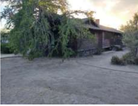
North face east side of building
