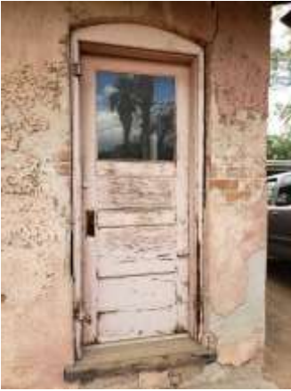
Example of original door
