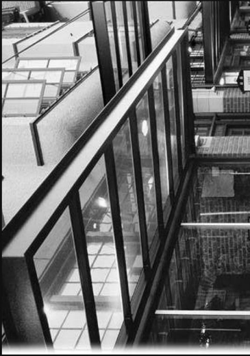
PAINTED STEEL CANOPY
