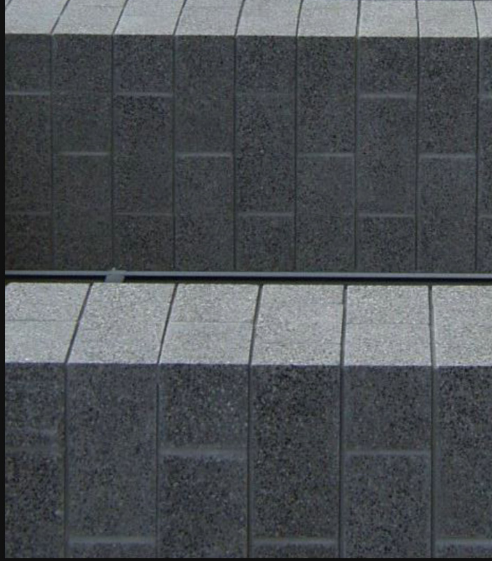
SHOT BLAST MASONRY
