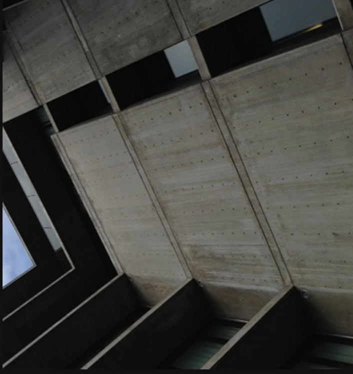
SITE CAST CONCRETE
