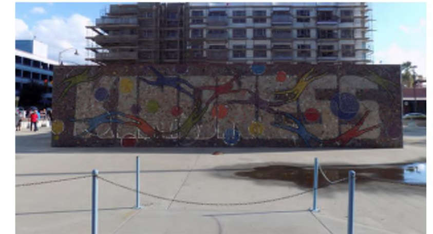
Tile Mosaic Wall 50' x 12' Salvaged from Existing Site Mounted on Steel Frame.
