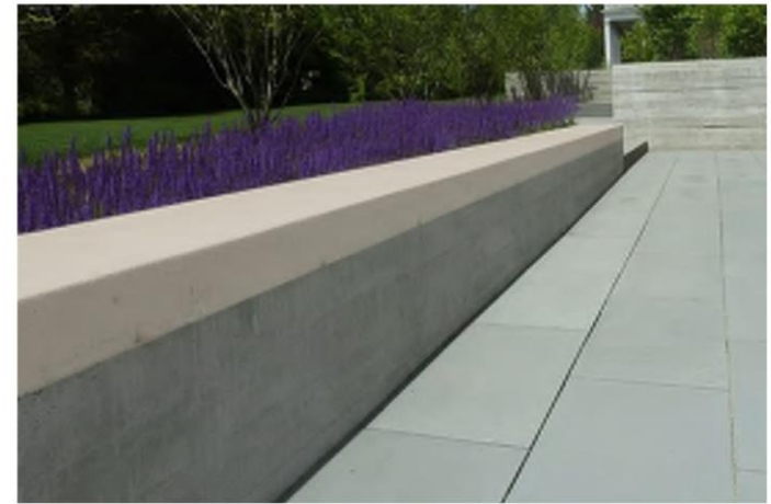
Seat Wall - Freestanding Concrete Cap Color: Scofield #C-12 Mesa Beige Primary Concrete Color: Scofield #C-34 Dark Gray
