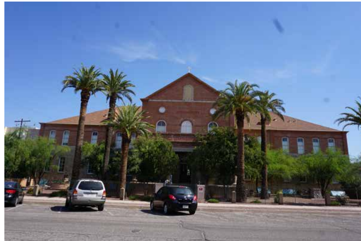
460 SOUTH 6TH AVENUE CONTIBUTING - LOCAL AND NATIONAL DISTRICT
