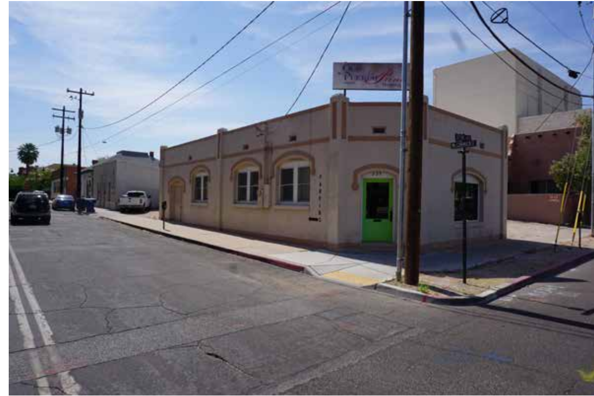
255 SOUTH STONE AVENUE CONTIBUTING - NATIONAL DISTRICT ONLY
