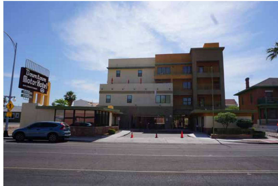
383 SOUTH STONE AVENUE CONTIBUTING - NATIONAL DISTRICT ONLY
