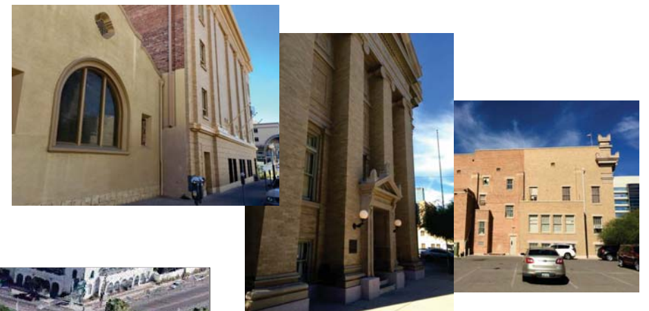
Scottish Rite Cathedral 160 S. Scott Ave. Historic Contributing Property
