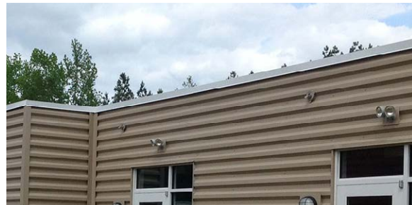
METAL PANEL PARAPET - ATAS
