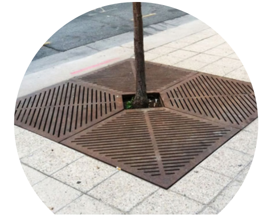
TREE GRATE WEATHERED STEEL
