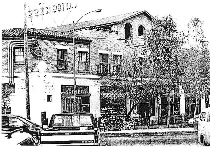
PHOTO #4: Partial view of north facade looking SW
