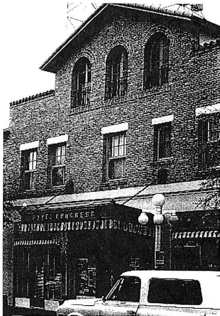
PHOTO #2: Congress Street façade detail of entry, looking NW
