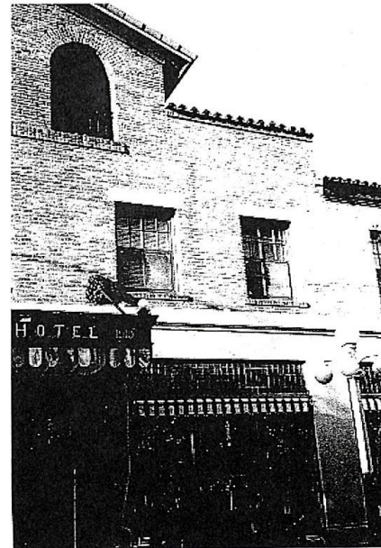
PHOTO #7: Detail of north facade showing ground floor storefront and second-floor facade zones; looking SW
