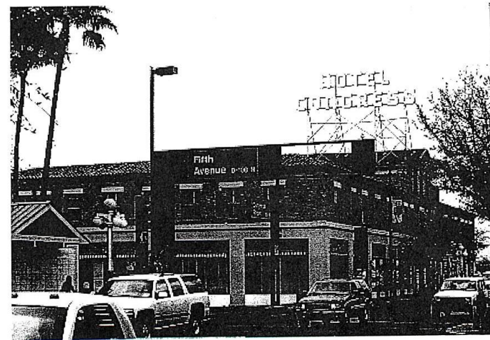
PHOTO #1: Three-quarter view of west and south facades from Congress Street; looking NE
