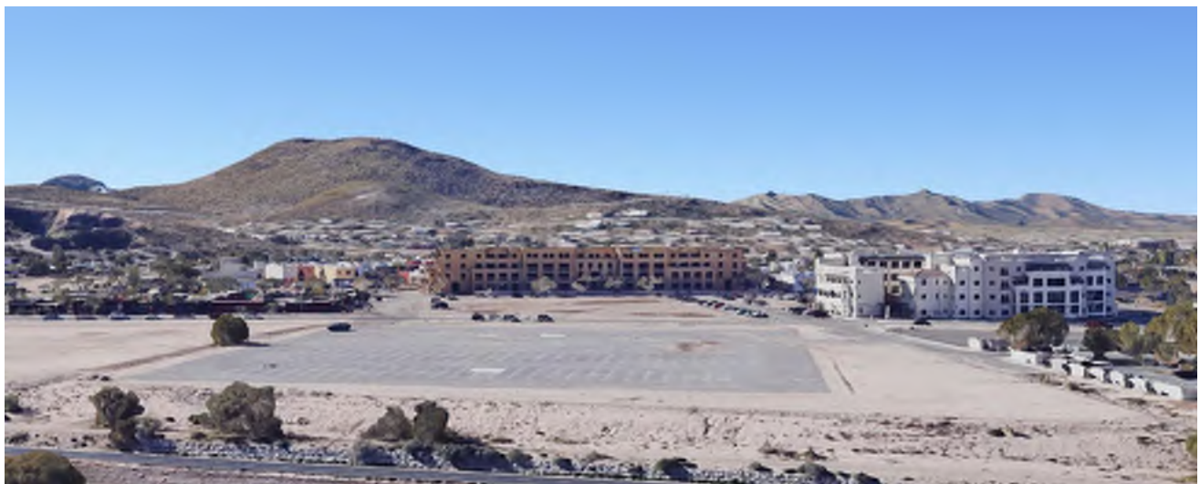
EAST ELEVATION – ARIEL
