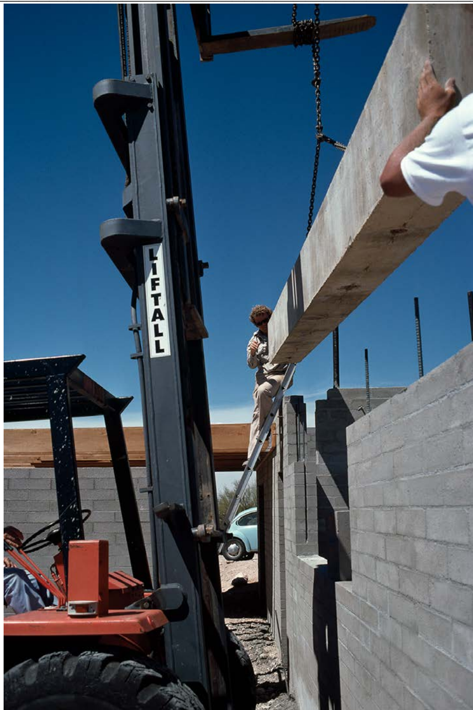
Fig 19. Jacobson House, construction photo, site cast concrete beam construction, 1977.
