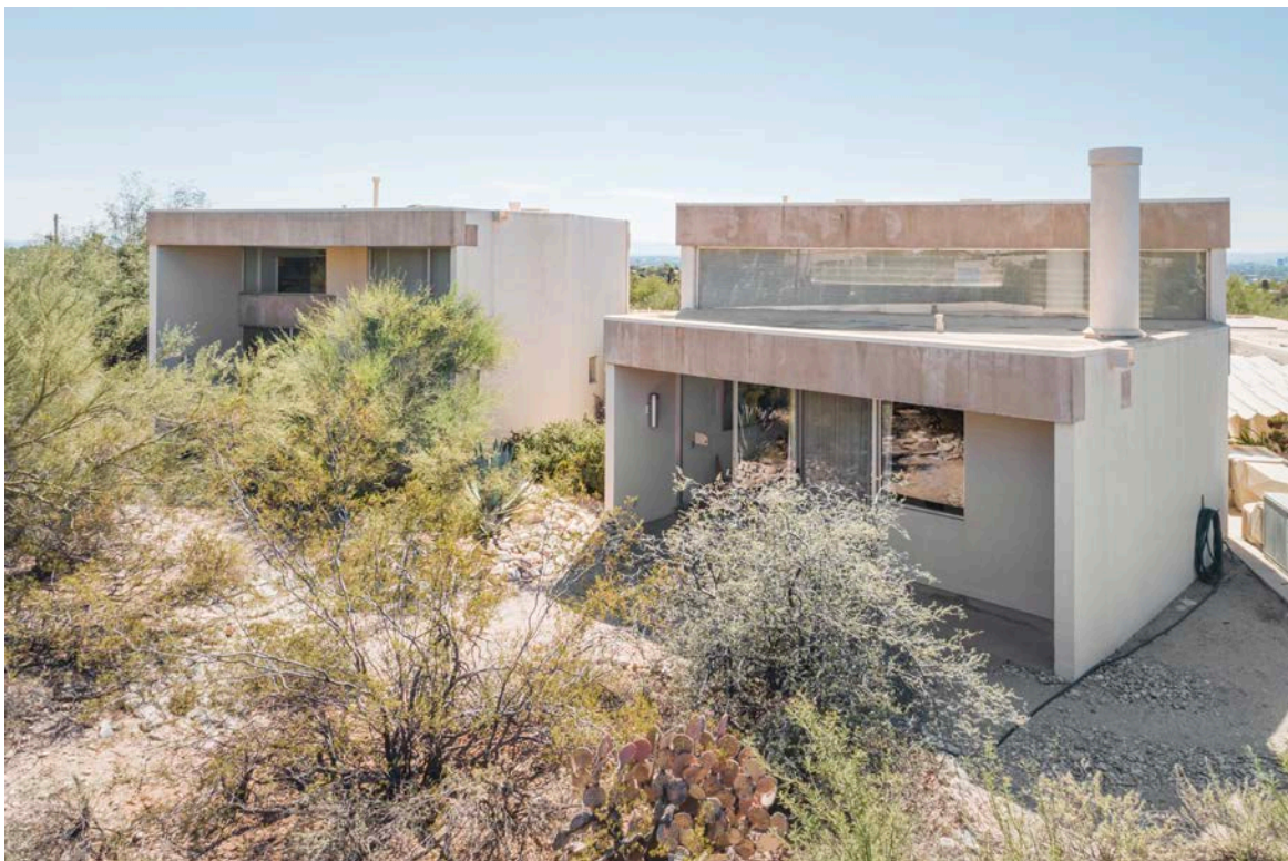
Fig. 4. North elevation, Massing, window system and clerestory windows. Photo GMVargas 2019.
