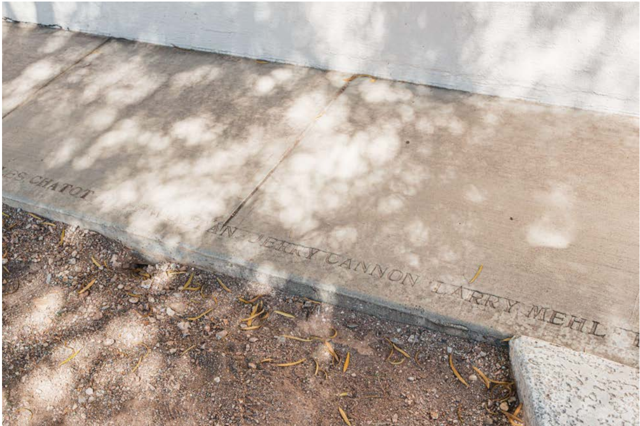
Photograph 11. Looking northwest, closeup, concrete walkway south facade. GMVargas.
