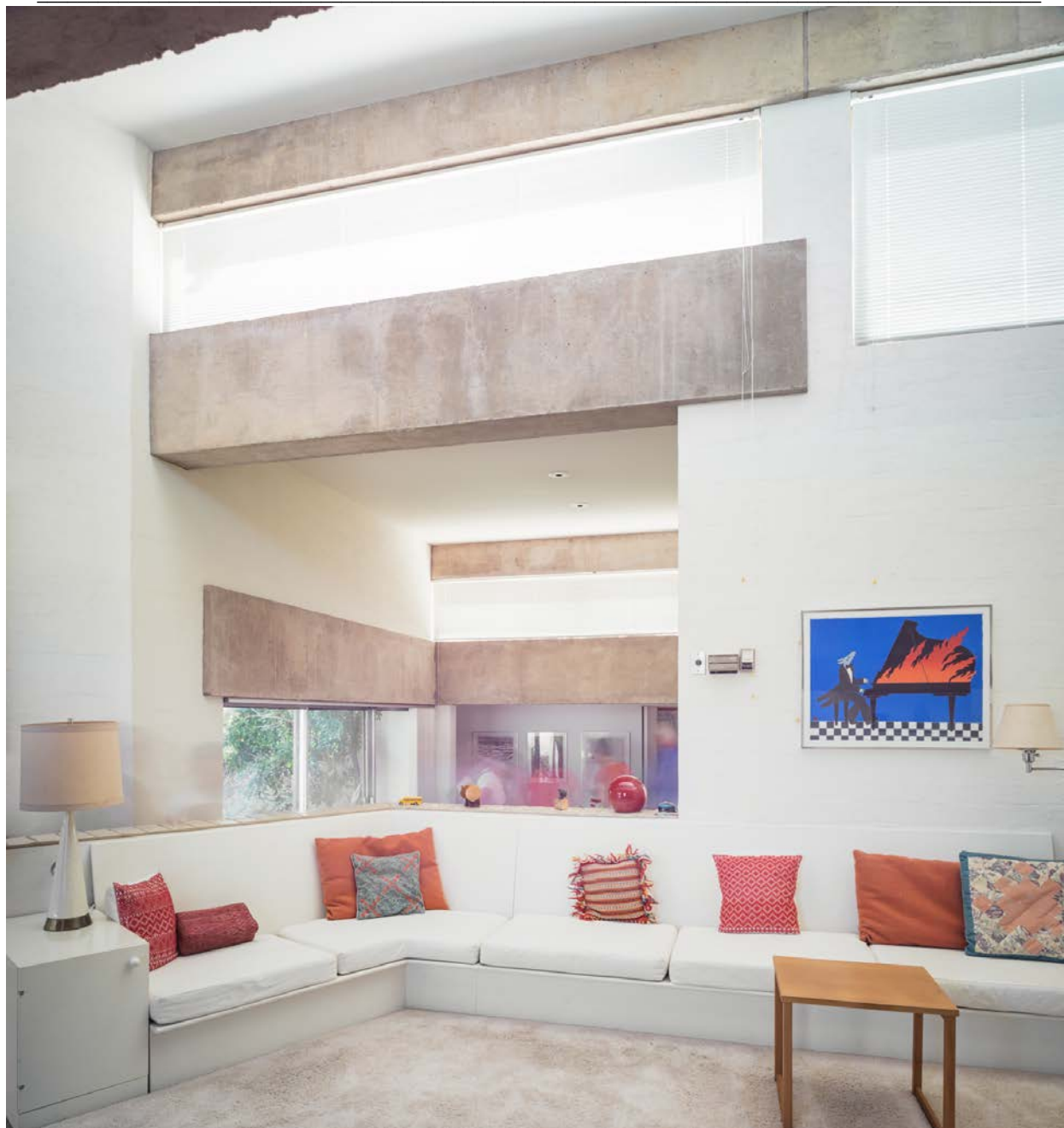
Fig. 11. Living room, cast concrete lenticils. Photo GMVargas 2019.
