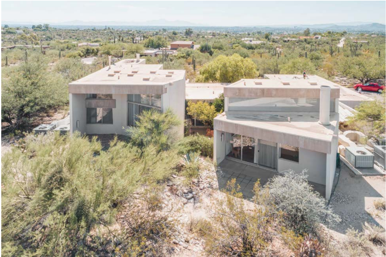
Photograph 3. Looking south, arial, north elevation. GMVargas.
