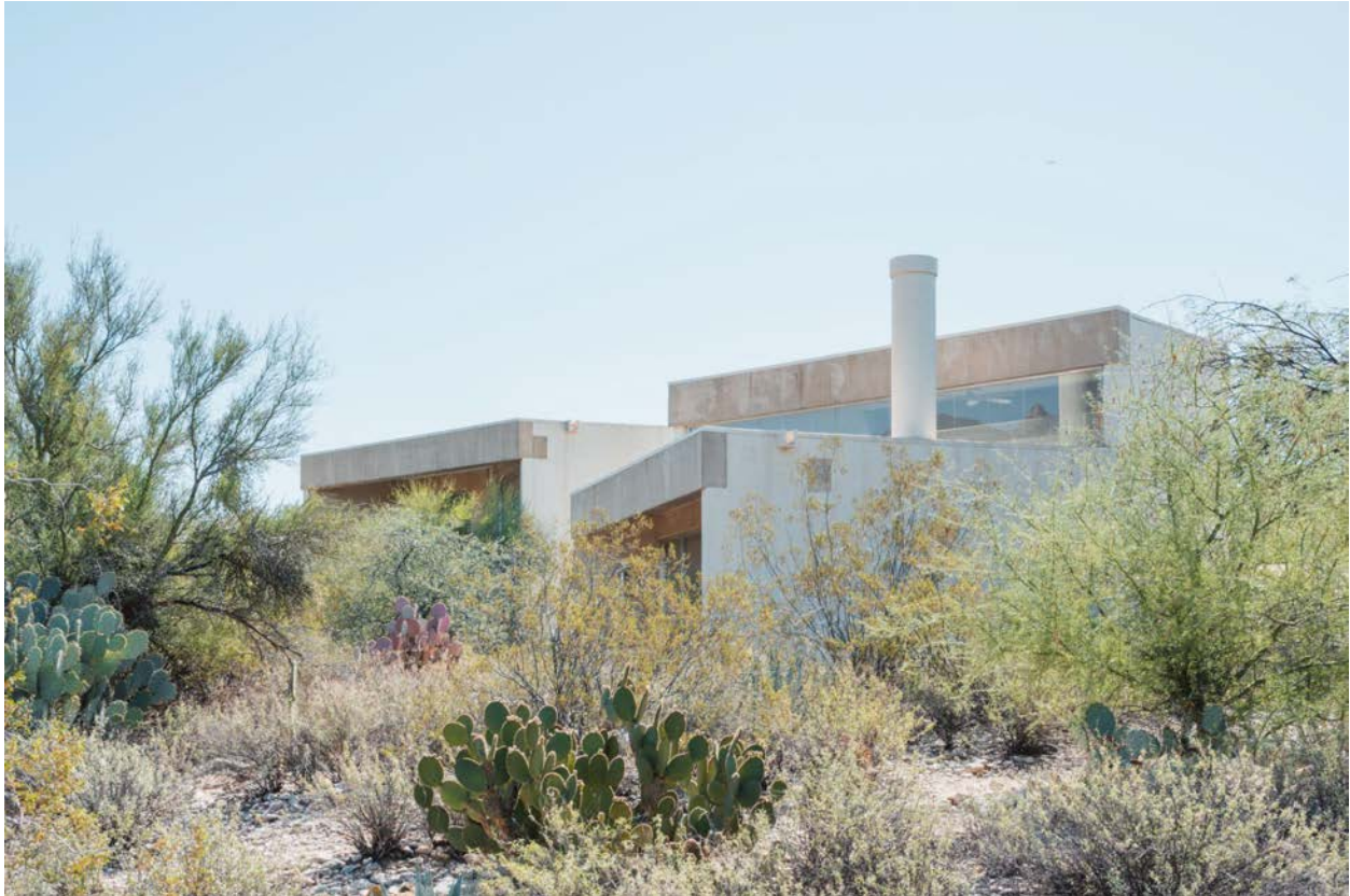
Photograph 1. Looking southeast, north elevation and desert site. GMVargas.
