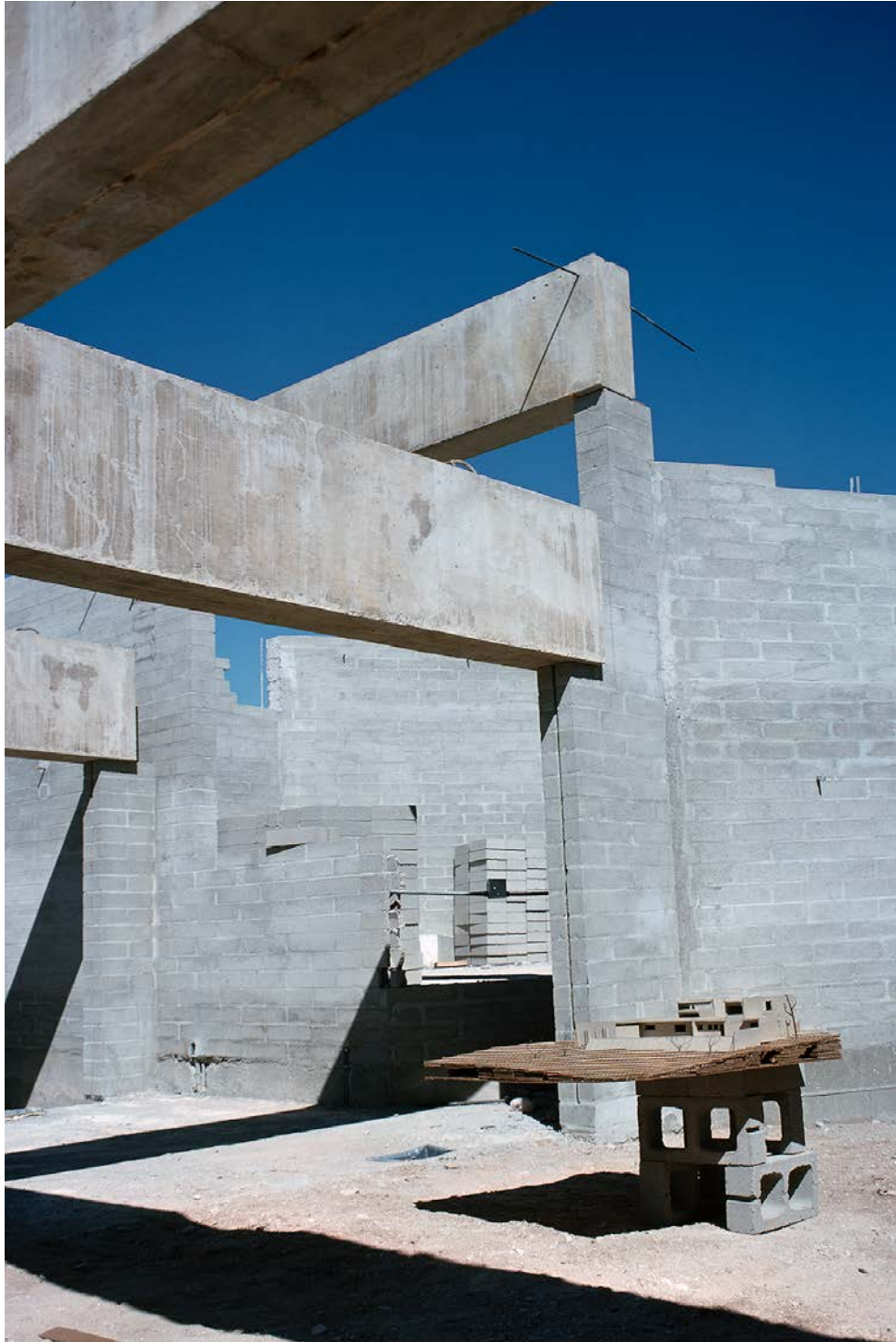
Fig 20. Jacobson House, construction photo, concrete beams and walls, 1977.
