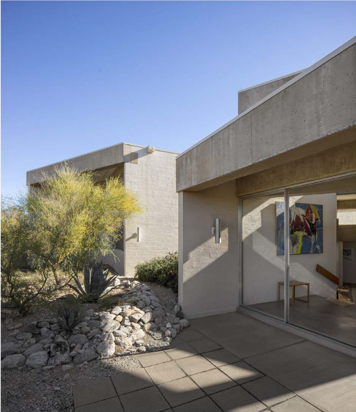
Photograph 7. Looking southeast, north elevation looking into the living room. Timmerman.
