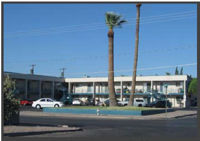
Two-Story Apartment Building
