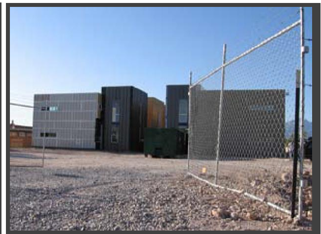
Infill Project Under Development
