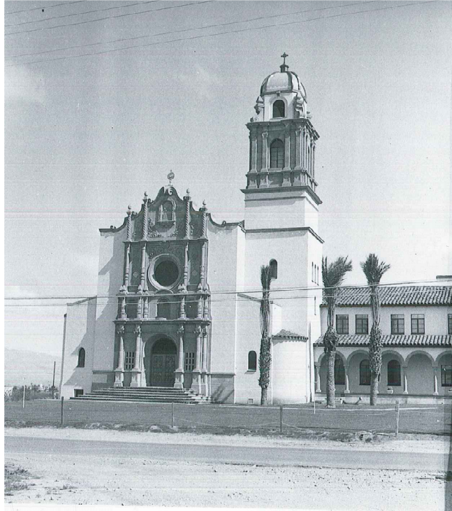
Figure 22. West façade with original date palms and lawn, ca. 1940s. Image courtesy of Arizona Historical Society (AHS No.75076)
