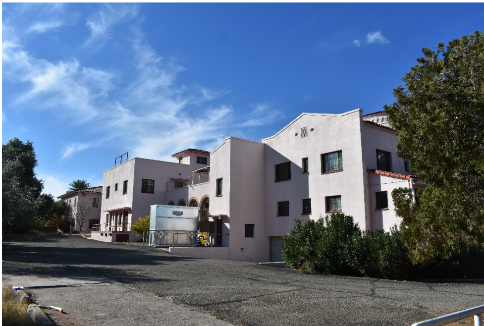
Figure 11. The east elevation of the Benedictine Convent and Chapel, facing southwest (2019).
