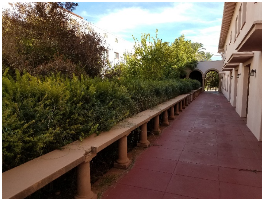
Figure 16. Walkway within the south courtyard, facing east-northeast (2019).
