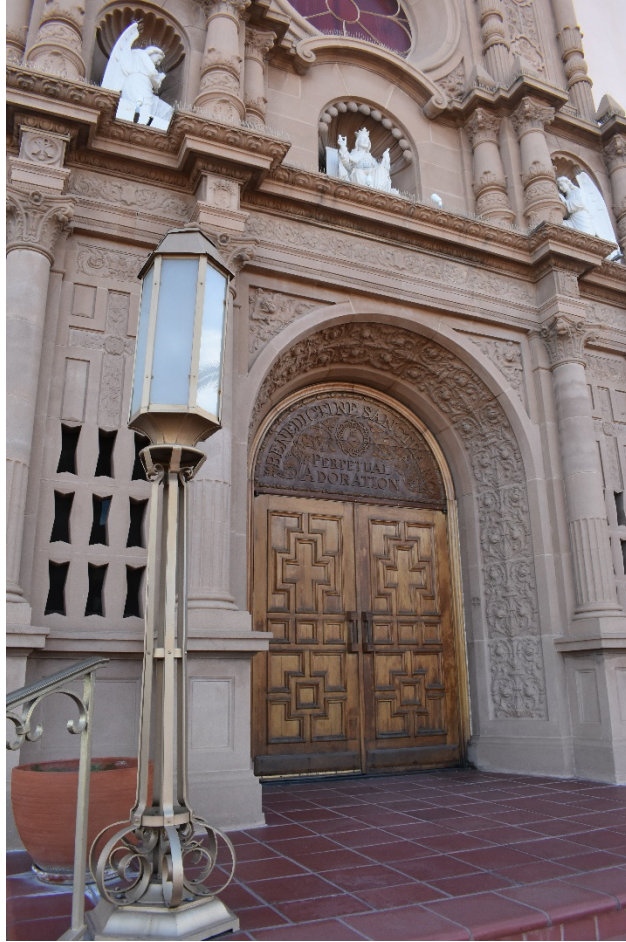
Figure 27. Entrance to sanctuary displaying a high-level of workmanship, facing southeast (2019).
