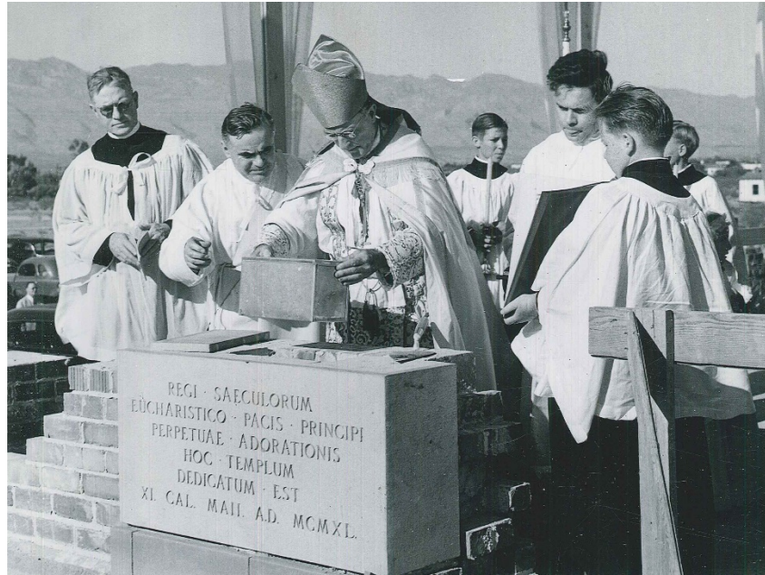
Figure 20. Laying of the cornerstone by Bishop Daniel Gerke, April 23, 1940. Image courtesy of Arizona Historical Society (AHS No. 7874).
