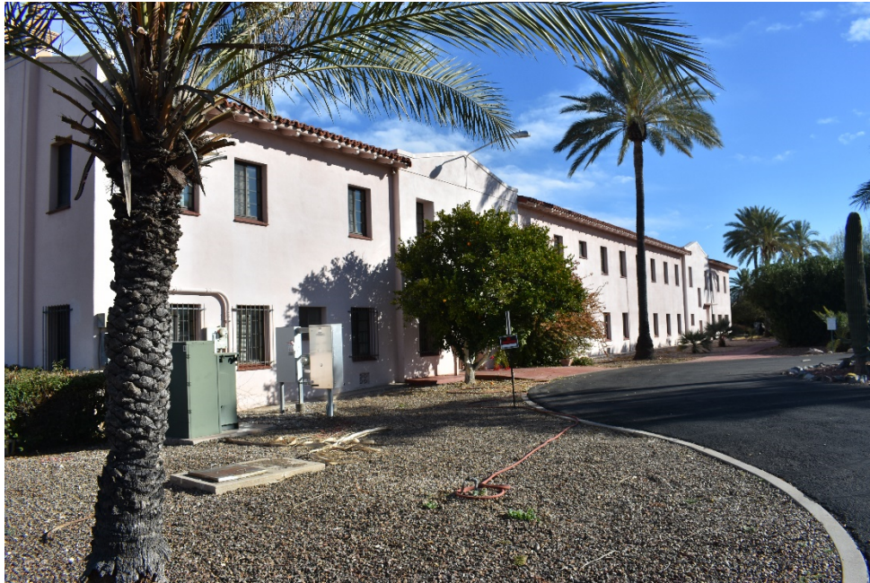
Figure 9. The south elevation of the Benedictine Convent and Chapel, facing northeast (2019).
