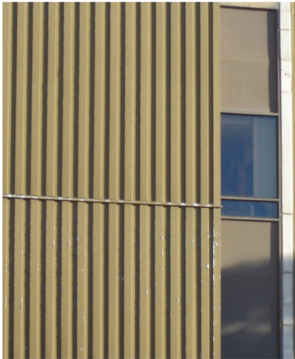
PRE-FINISHED METAL PANELS, ALUMINUM STOREFRONT
