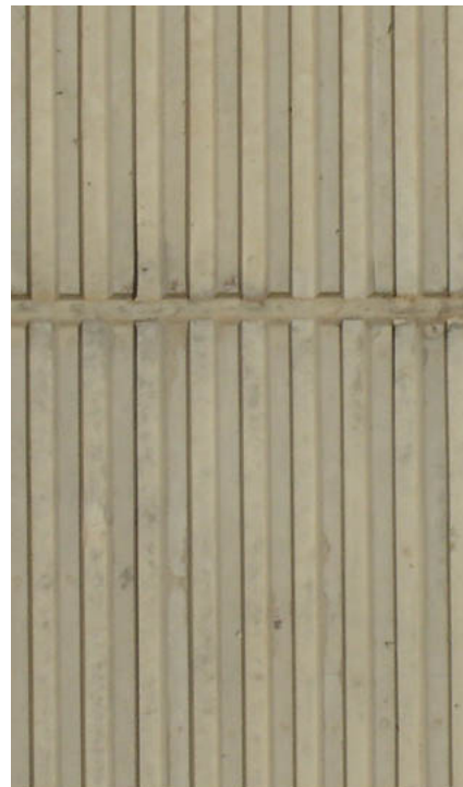
CAST-IN-PLACE CONCRETE RIBBED FORM TEXTURE
