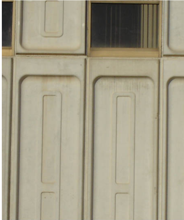
PRE-CAST CONCRETE PANELS, ALUMINUM STOREFRONT & TINTED GLASS
