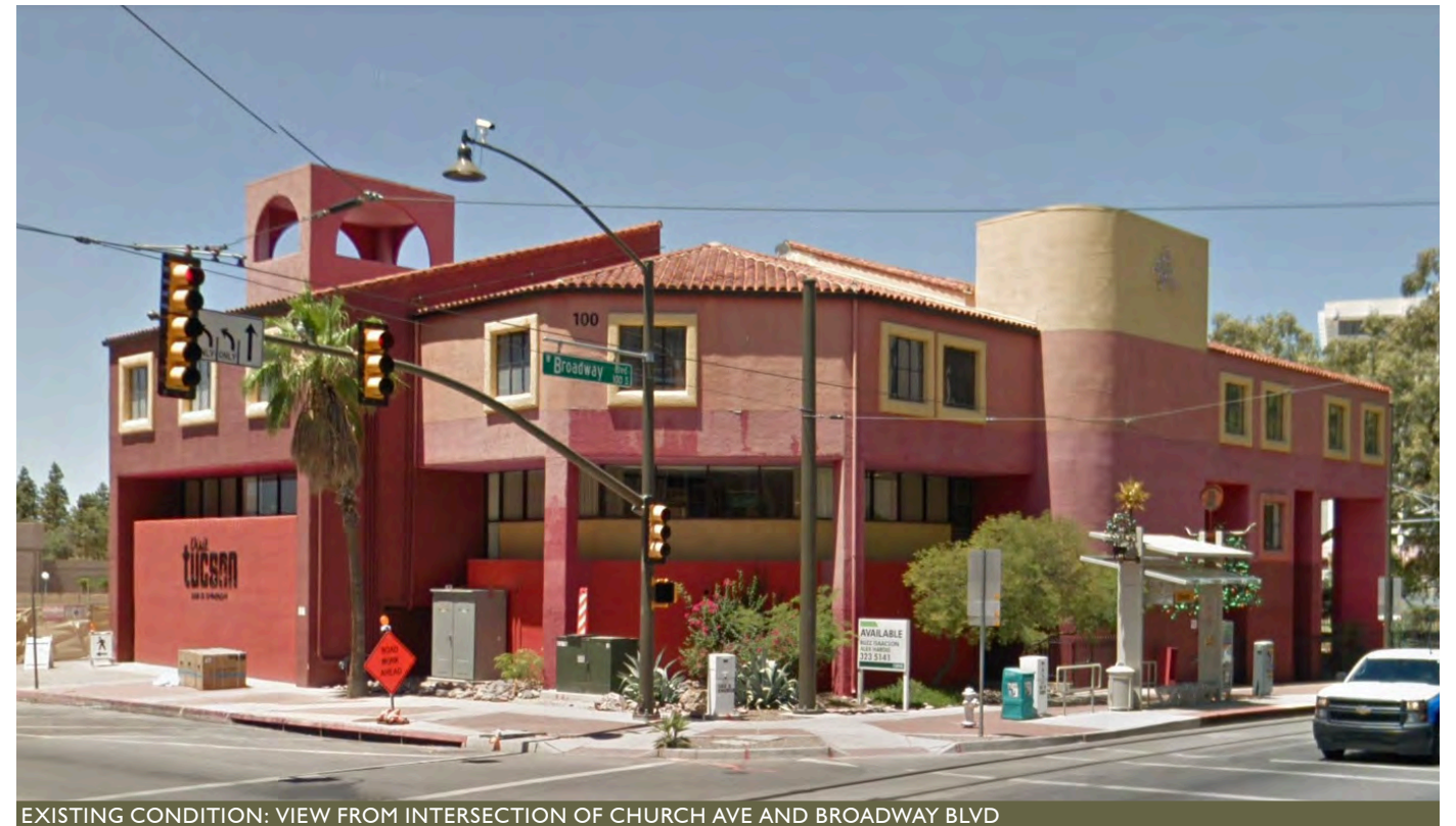
EXISTING CONDITION: VIEW FROM INTERSECTION OF CHURCH AVE AND BROADWAY BLVD
