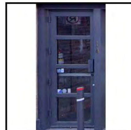
DOOR TO MATCH EXISTING HIGHWIRE WITH ARCHED WINDOW ABOVE
