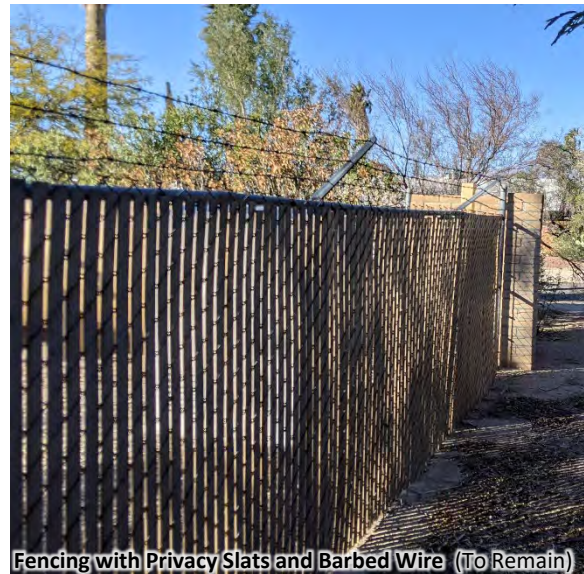
Fencing with Privacy Slats and Barbed Wire (To Remain)
