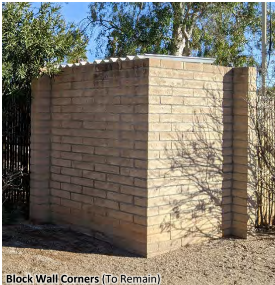
Block Wall Corners (To Remain)
