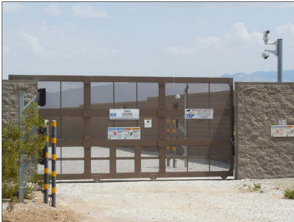
Photo 1. Example Substation Signage
