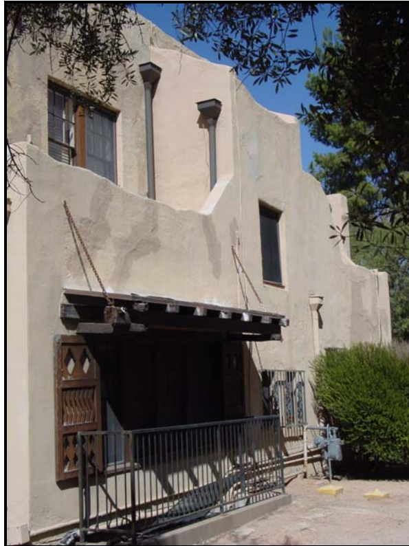
Photograph 28. Detail of east elevation of Erickson Residence, looking northeast (2009).
