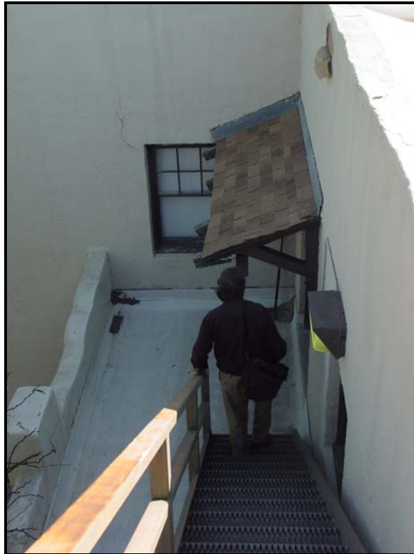
Photograph 21. Second-story porch and roof access on east elevation, looking south (2009).
