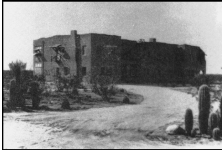
Photograph 15. Historical photograph of the Arizona Building (Nurses' Residence) looking west-northwest, 1927 (courtesy of Tucson Medical Center).
