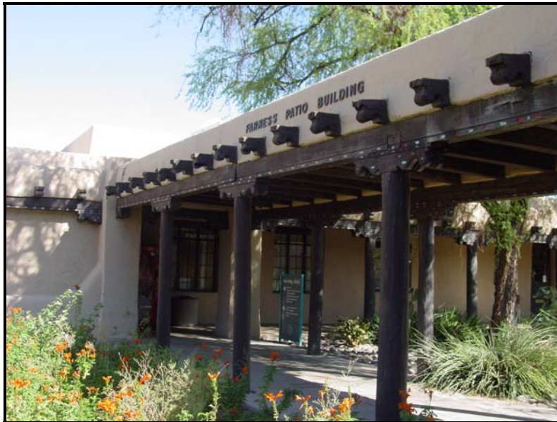
Photograph 8. Detail of west elevation loggia of the Patio Building, looking north (2009).
