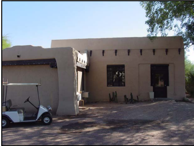
Photograph 9. Southwest corner of the west elevation of the Patio Building, looking east (2009).
