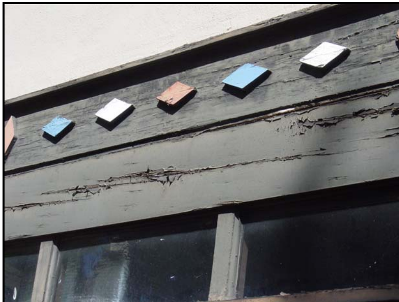
Photograph 19. Detail of wood headers along south elevation of the Arizona Building (2009).
