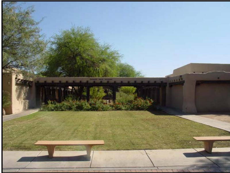
Photograph 7. West elevation of the Patio Building, looking east (2009).
