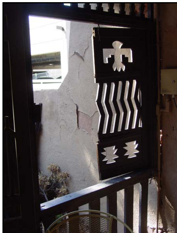
Photograph 33. Detail of porch shutters on the Erickson Residence, looking west (2009).
