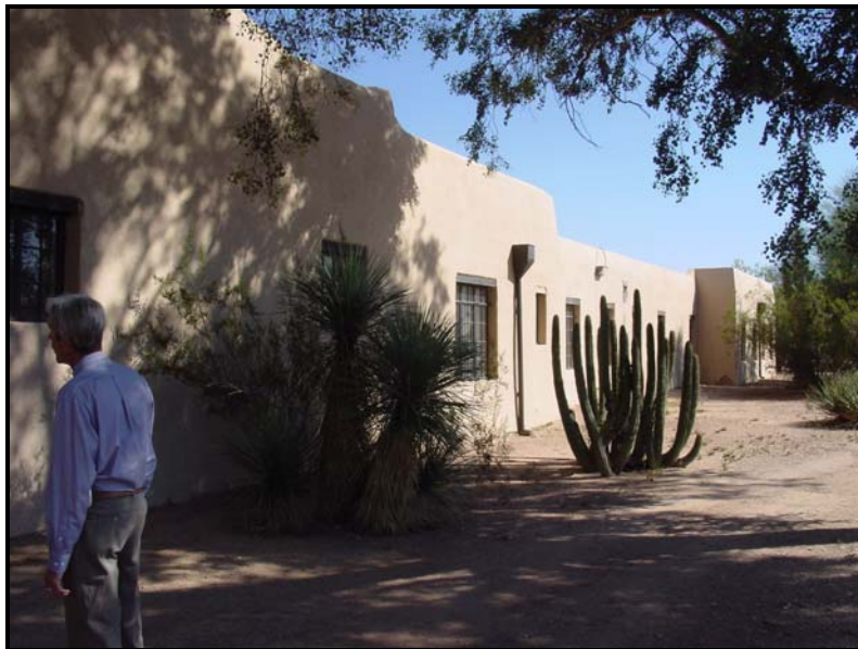
Photograph 14. South elevation of the Patio Building, looking east (2009).
