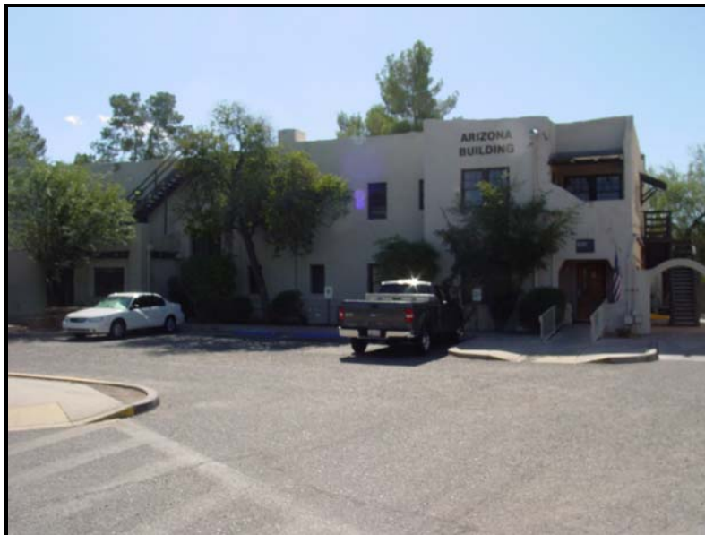
Photograph 16. East elevation of the Arizona Building, looking west-southwest (2009).
