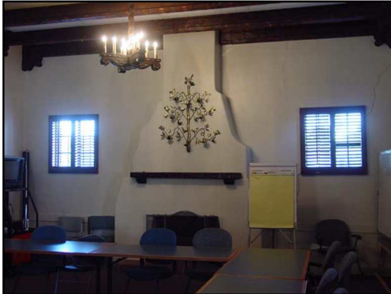
Photograph 13. Interior of reception room (now conference room) of the Patio Building, looking south (2009).
