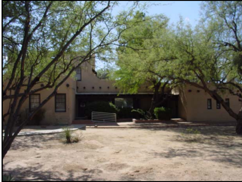
Photograph 26. North elevation of the Erickson Residence, looking west (2009).
