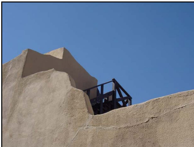
Photograph 29. Detail of roofline and porch along east elevation of the Erickson Residence (2009).
