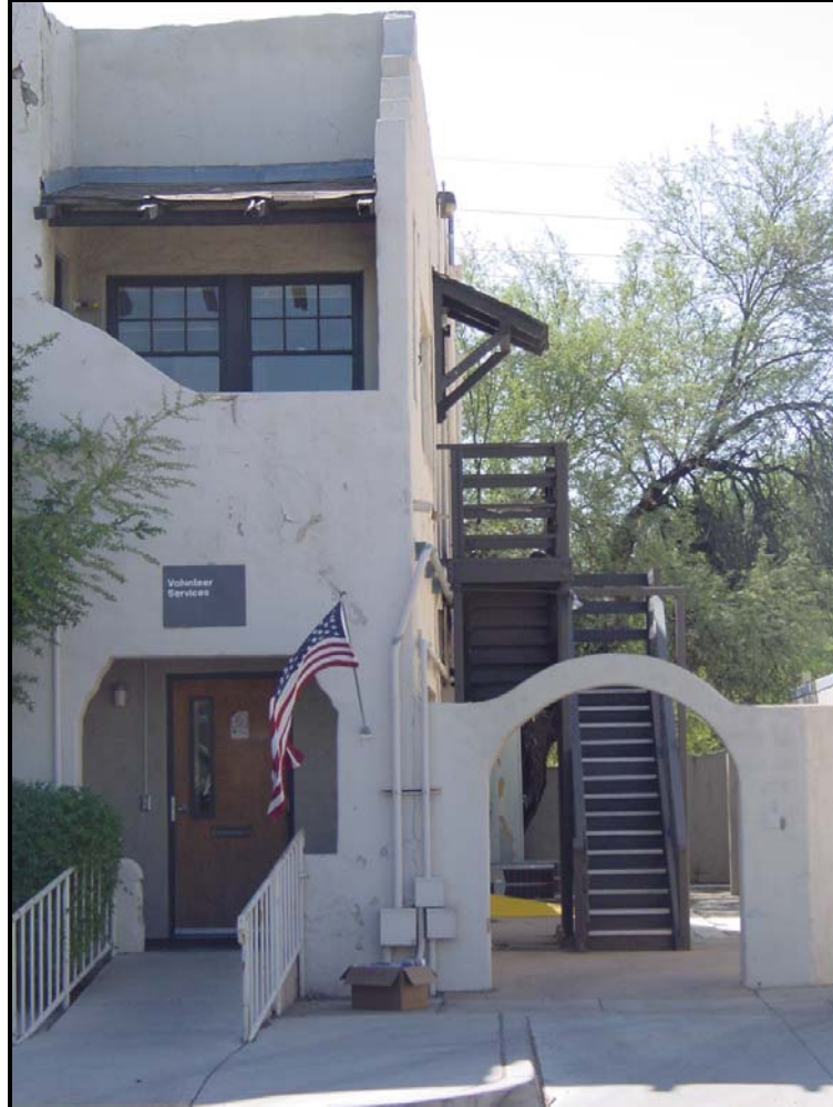
Photograph 17. Detail of northeast corner of the Arizona Building, looking west (2009).
