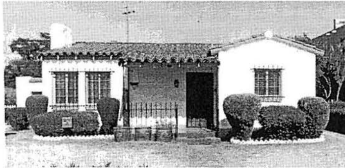
This simple ca. 1939 house illustrates the transition from the Period Revival to post-World War II tract houses. The basic plan of the Ranch Style (or Minimal Traditional) can be detected while it still conveys the flavor of Spanish Colonial Revival.
